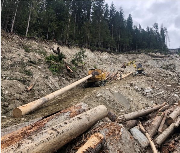
Figure 12 - Log supply by tracked vehicle along temporary access road. Photo by McElhanney (July 25, 2020).
