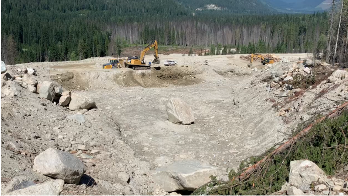
Figure 5 - Excavation of MRB
