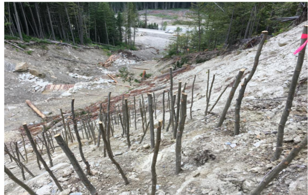
Figure 15 - Live-staking of gully side slopes. Photo by Brinkman Restoration. (August 31 – September 2, 2020)
