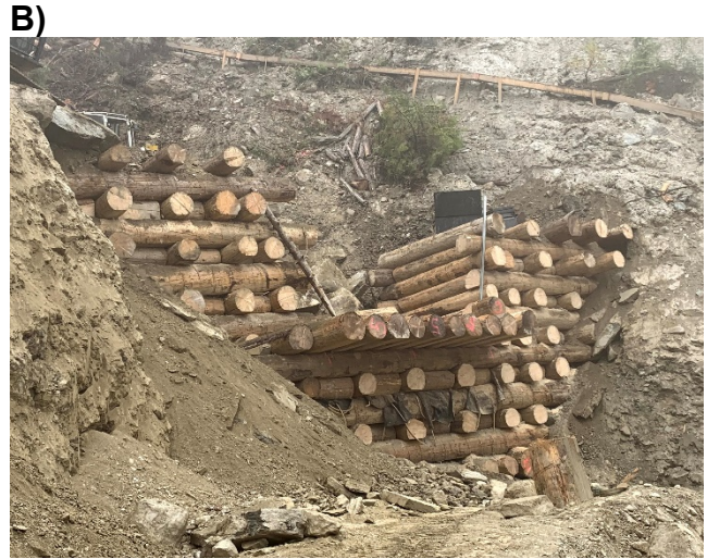
Figure 17 A) Front face abrasion observed after the 2021 freshet (Photo by Pierre Friele). B) New check dam built in 2021 with overhang to protect front face from abrasion (Photo by McElhanney)
