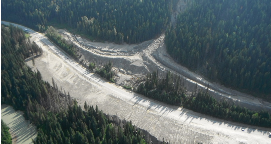
Figure 2 - View from Helicopter looking northeast at moustache-shaped retention basins (MRB) protecting the Trans-Canada Highway (TCH). Note: some of the debris excavated from the MRB is deposited between the TCH and the Beaver River (Photo by Tetra Tech EBA, 2014).
