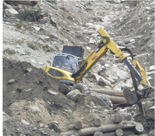
Figure 19 A) Damage to Check Dam 5 caused by the Lateral landslide. B) Construction of sill log structures to stabilize the thalweg.
