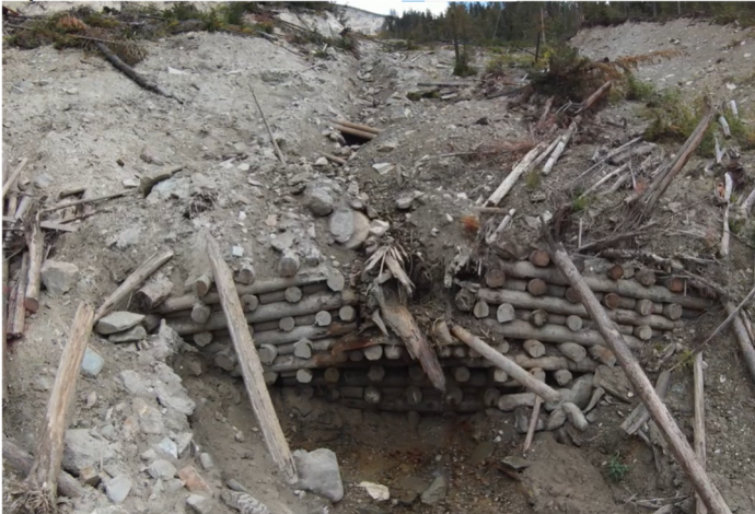
Figure 19 A) Damage to Check Dam 5 caused by the Lateral landslide. B) Construction of sill log structures to stabilize the thalweg.
