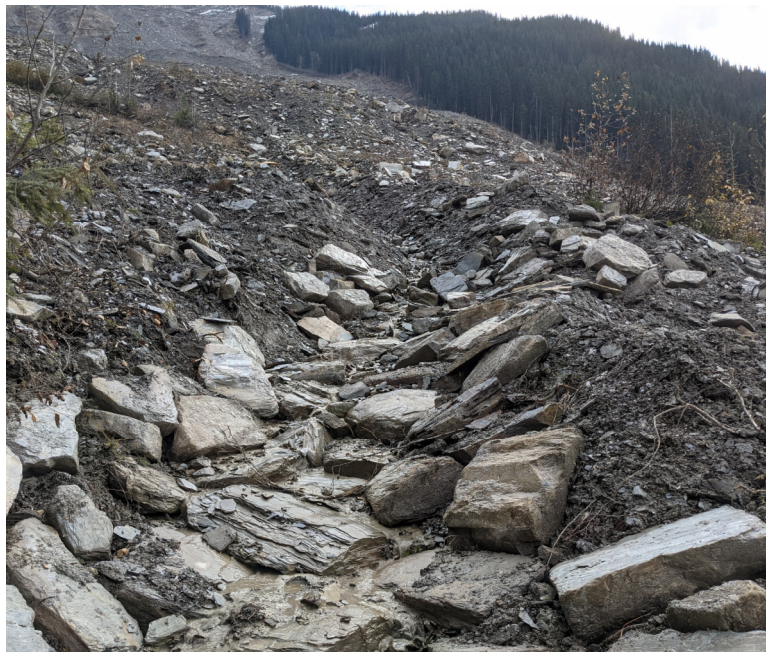
Figure 20 Drainage diversion in the upper catchment area
