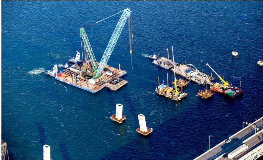
Figure 20: Installation of Underwater Foundations at Competent Rock
