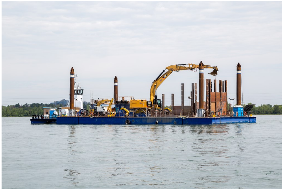
Figure 14: Excavation Barge and Dredging Barge
