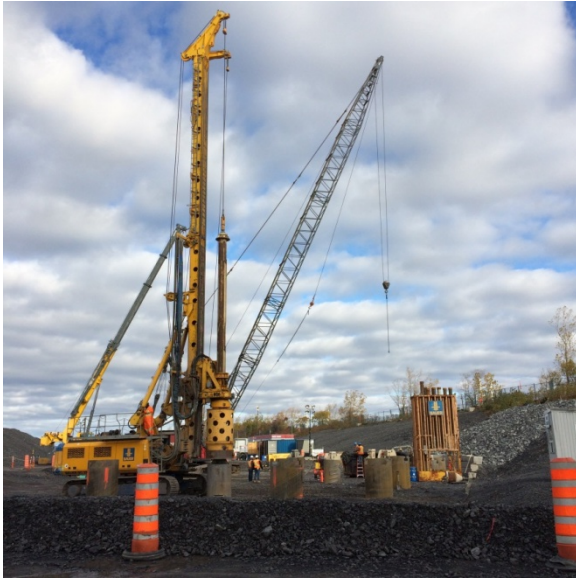
Figure 12: Drilling of caissons
