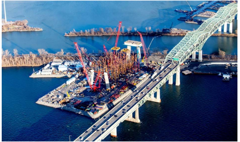
Figure 13: Construction of the Main Pier
