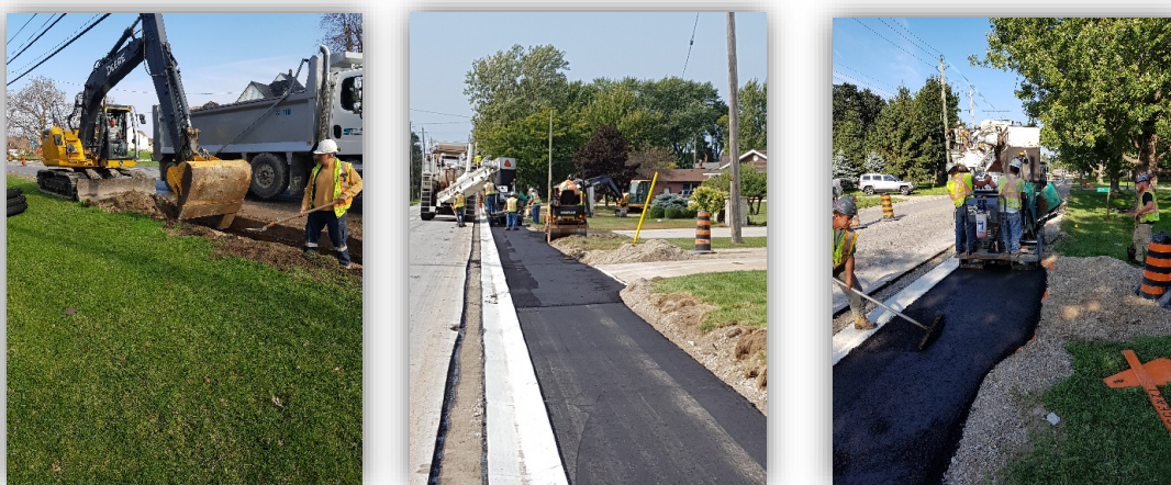
FIGURE 6: PHOTOS DURING CONSTRUCTION OF THE COUNTY ROAD 20 ONE-WAY CYCLE TRACK
