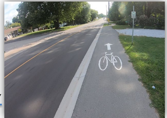
Completed Cycle Facility
