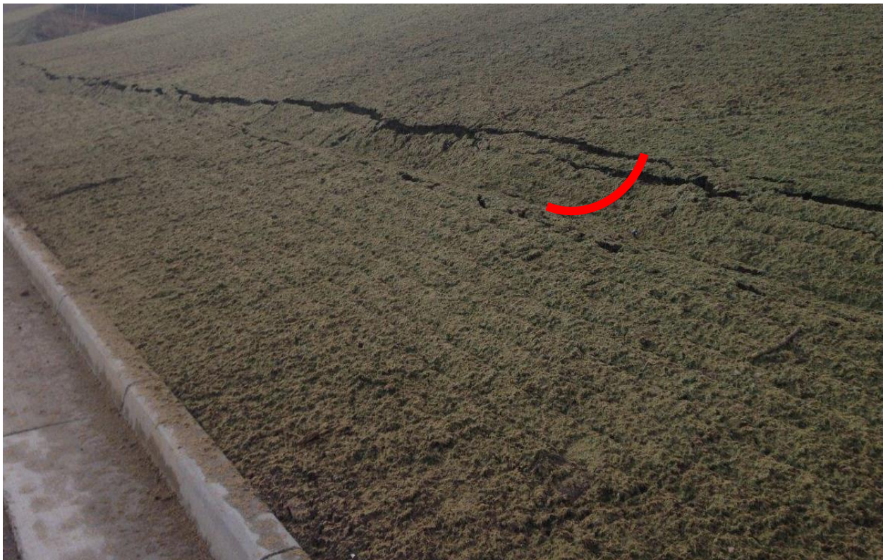
Figure 2. Cross-gradient water bar graded swale soil texturing
