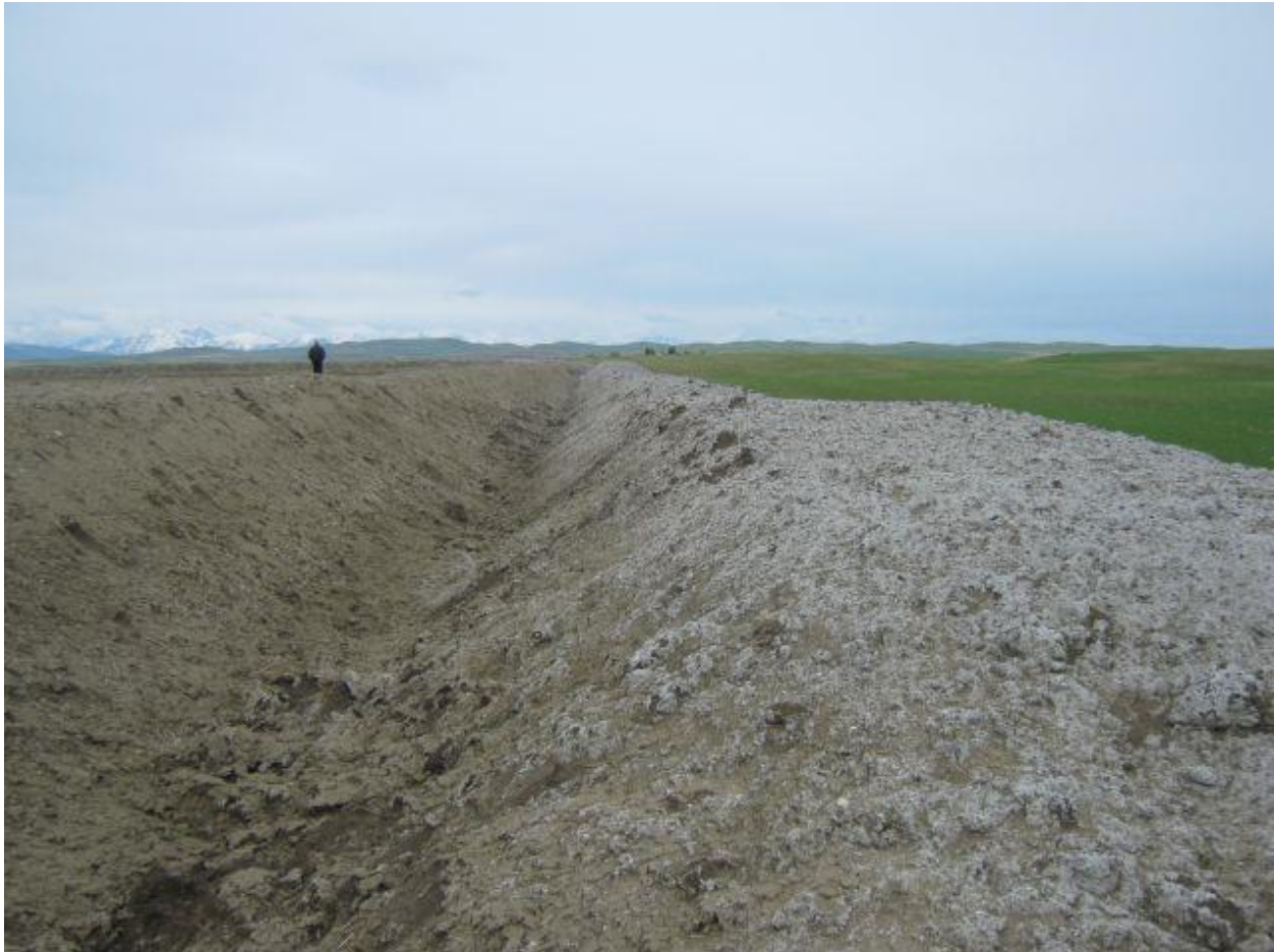
Figure 7. Highly conforming Hydraulically Applied Erosion Control mulch high wind performance
