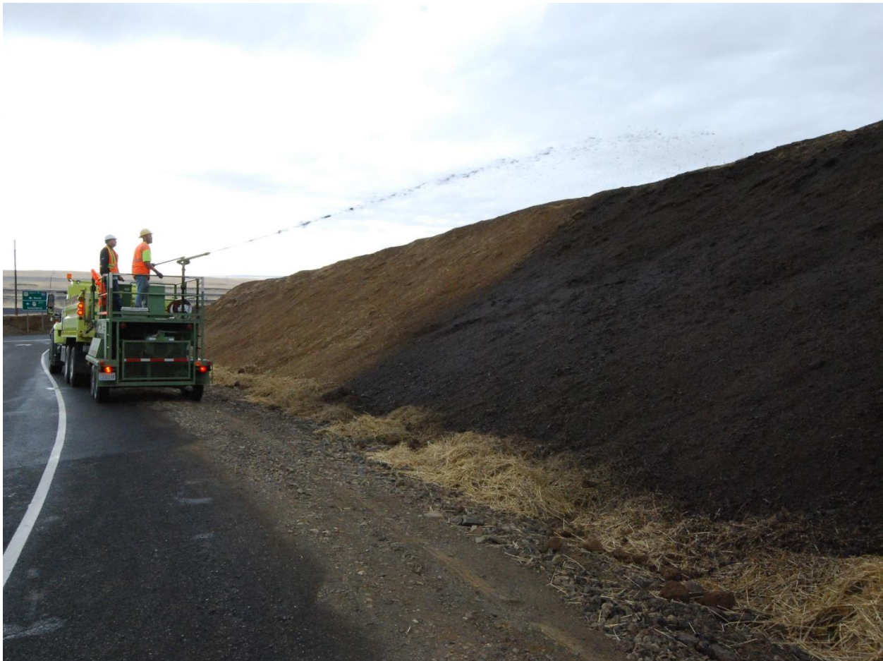
Figure 8. Hydraulically Applied Biotic Soil Amendment (HBSA)
