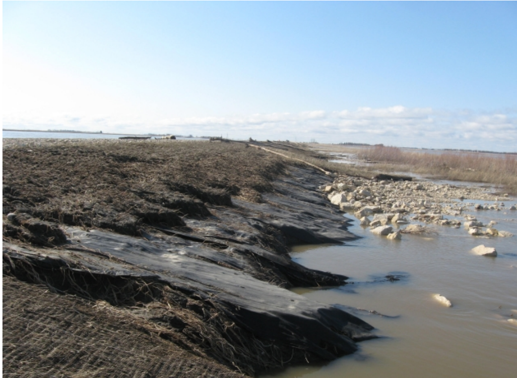
Spring, 2009 300mm rock armour conveyed in overtopping, adjacent TRM in the foreground performed
