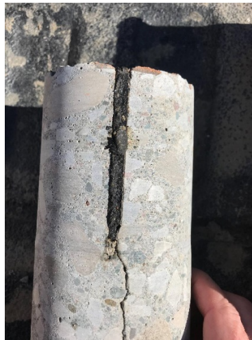
Figure 8: Core at the Joint Filled with Sealant
