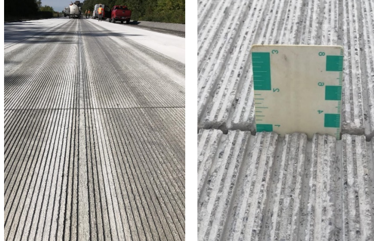
Figure 7: Final Diamond Grinding and Grooving Texture
