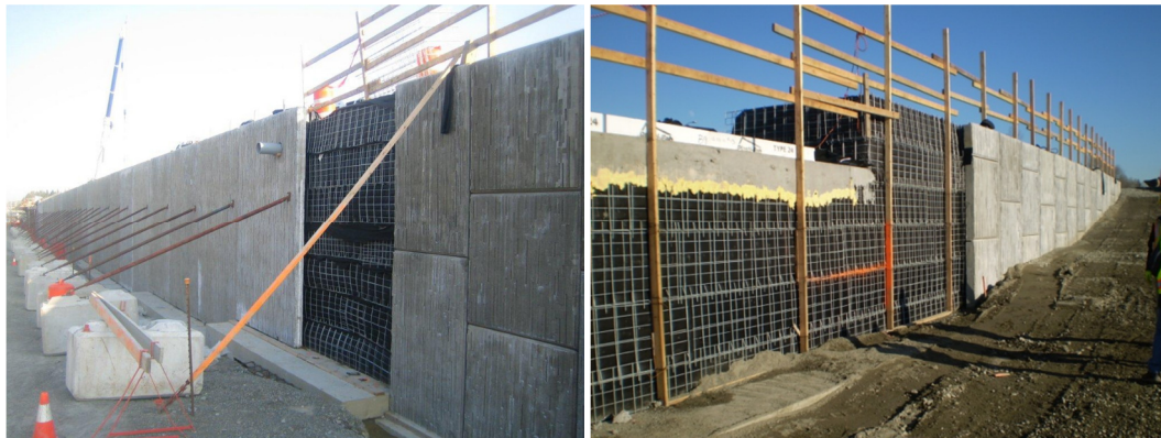
Figure 18 – EPS to MSE Transition at 202 nd Street EPS Embankments
