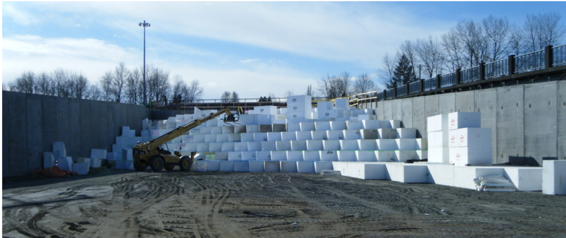
Figure 3 – Placement of Blocks at Kensington Avenue EPS Embankment
