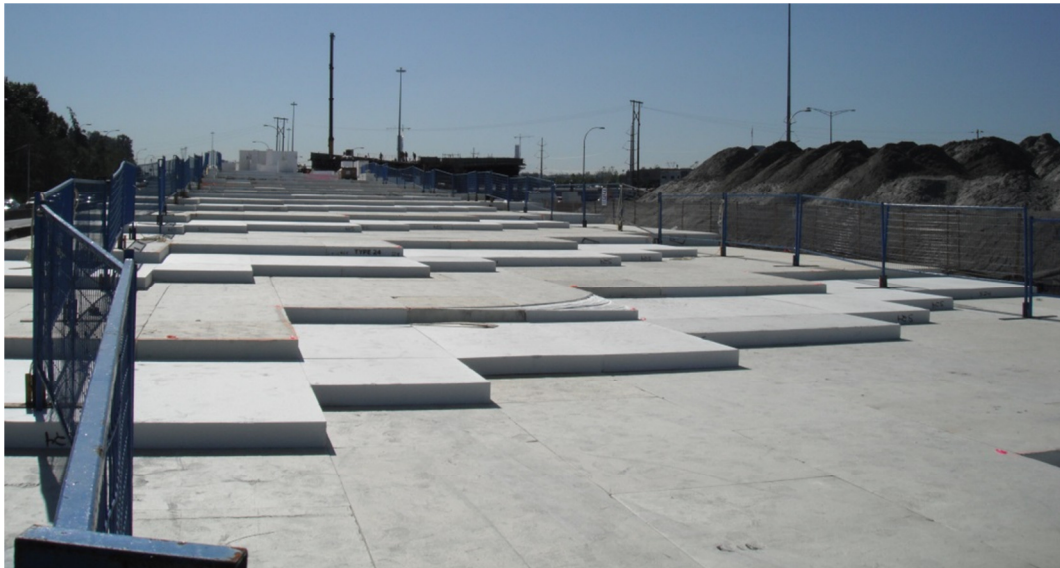
Figure 8 – Top Surface of EPS Blocks at E5901N EPS Embankment
