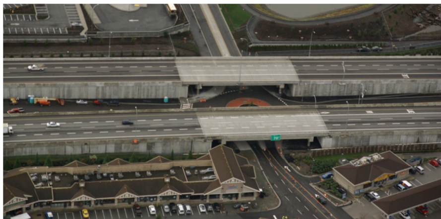
Figure 16 – Aerial View of Completed 202 nd Street Overpasses and EPS Embankments
