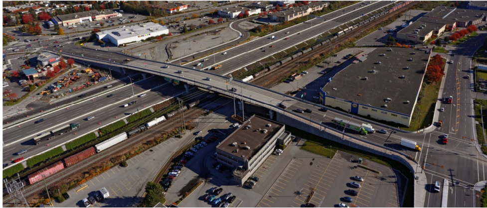
Figure 15 – New King Edward Overpass
