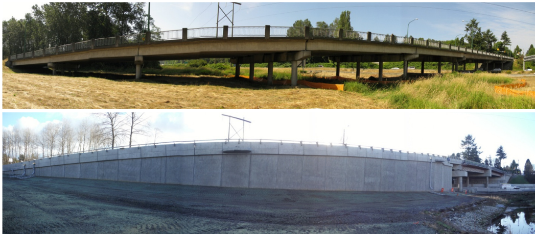
Figure 13 – Original Sprott Street Overpass (top) and New EPS Embankment (bottom)
