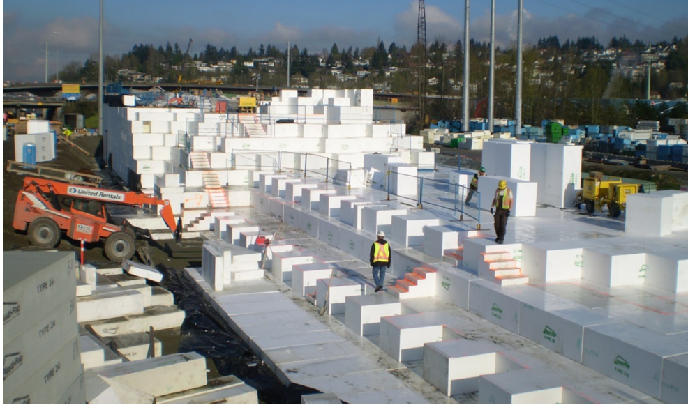
Figure 2 – EPS Embankment Under Construction
