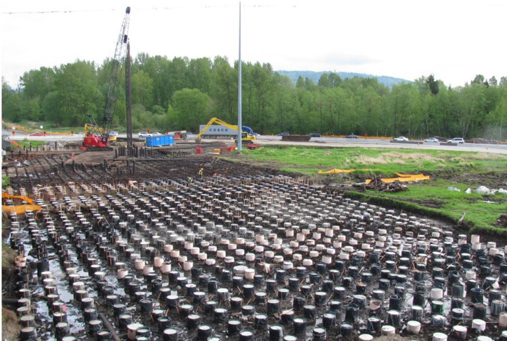
Figure 6 – Timber Pile Installation at Kensington Avenue EPS Embankment
