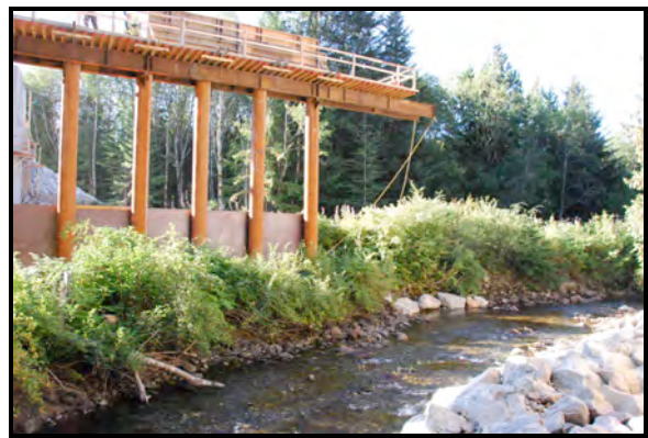
Figure 7: New bridge at Millar Creek
