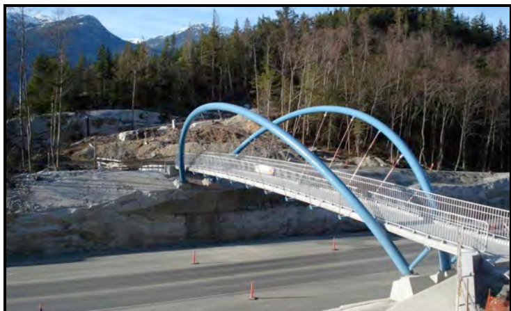
Figure 9: Stawamus Chief pedestrian bridge
