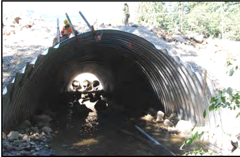
Figure 5: Bottomless culvert replacing 3 round culverts at Widow Cr.
