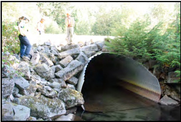
Figure 6: Existing culvert at Millar Creek
