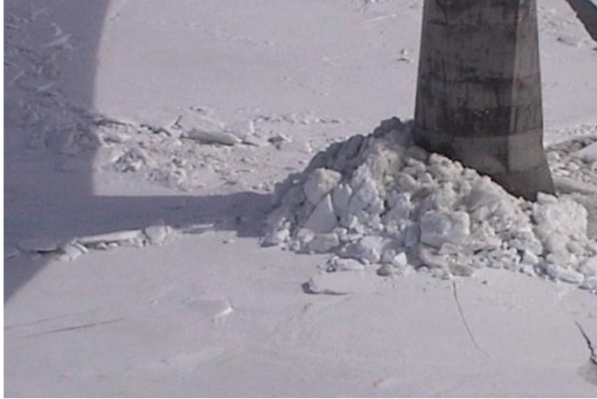
Figure 6 Typical Rubble Pile
