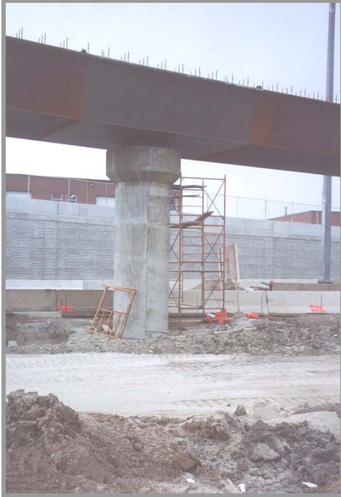
Single Pier with single bearing
