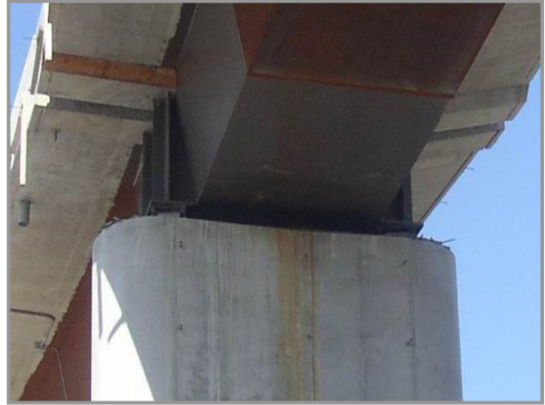
Wide diaphragm at Bridge 205
