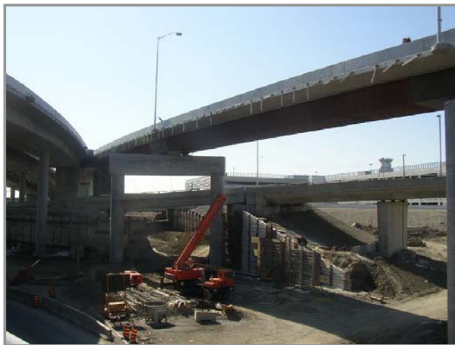
Pier 1 of Bridge 311
