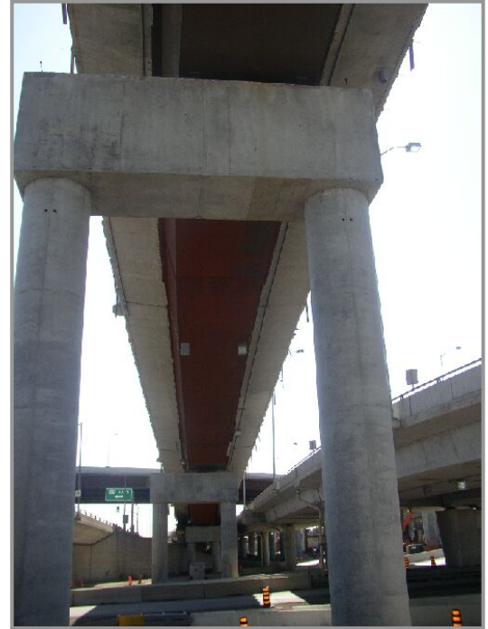
Piers 3 and 4 of Bridge 205
