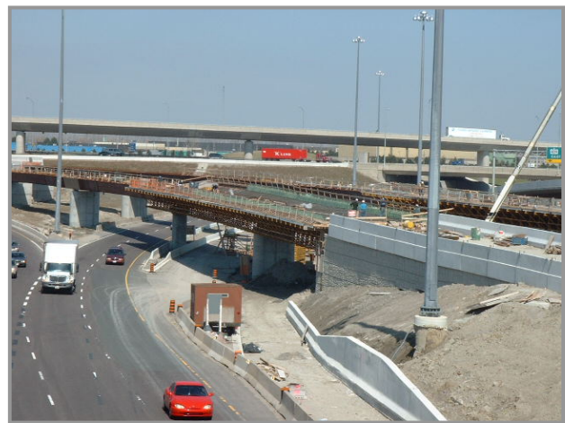
Deck construction of Bridge 604
