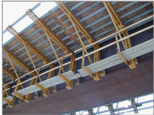
Falsework for deck cantilever
