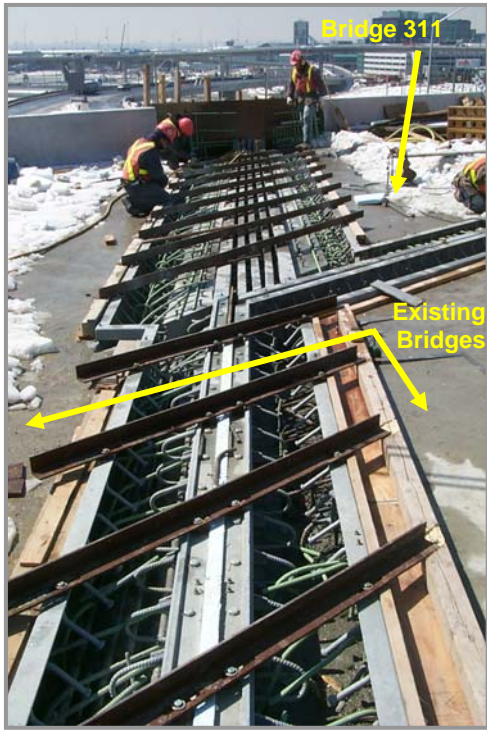
Expansion joint of Bridge 311
