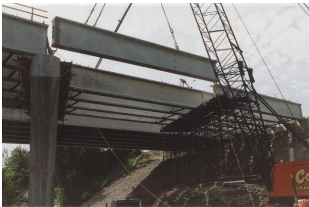
(a) Girder erection using temporary bents
