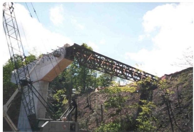
(b) Girder erection using a launching truss
