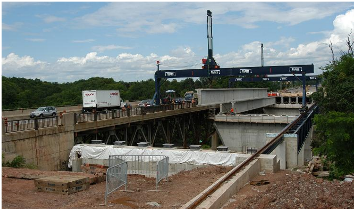
Figure V: Overhead gantry for lifting and placing field spliced precast concrete girders
