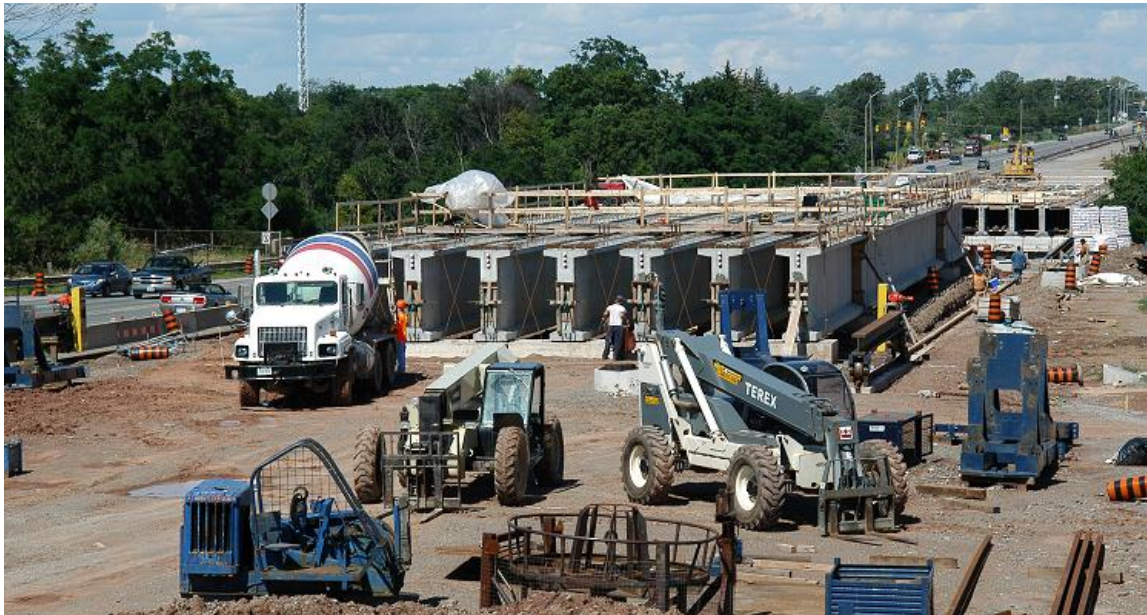
Figure VI: Splicing bed for joining precast concrete girder segments on-site
