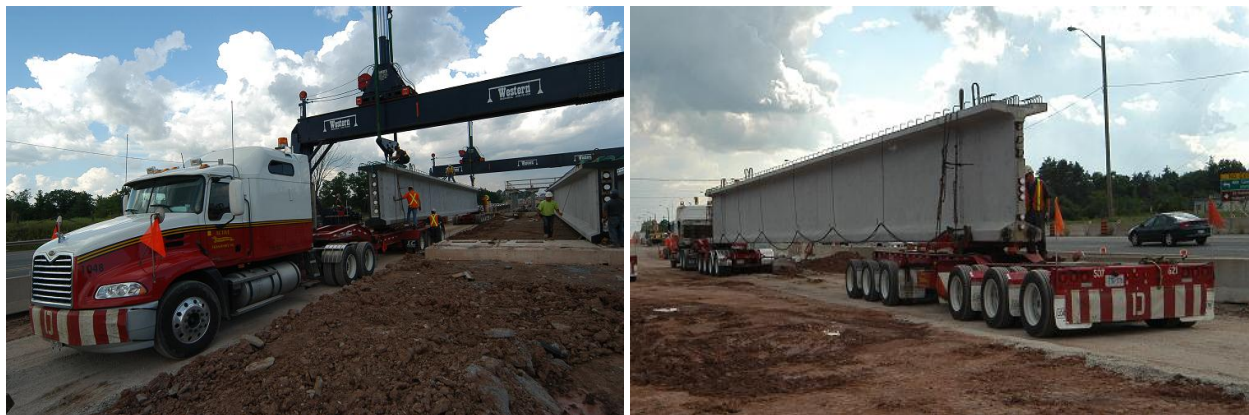
(a) Semi-tractor with jeep to support girder
