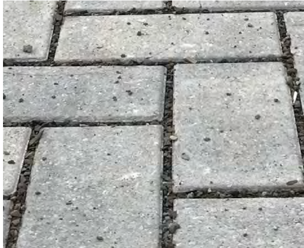
Figure 3-5: Visual inspection of the PICP joints after the third round of clogging before compaction
