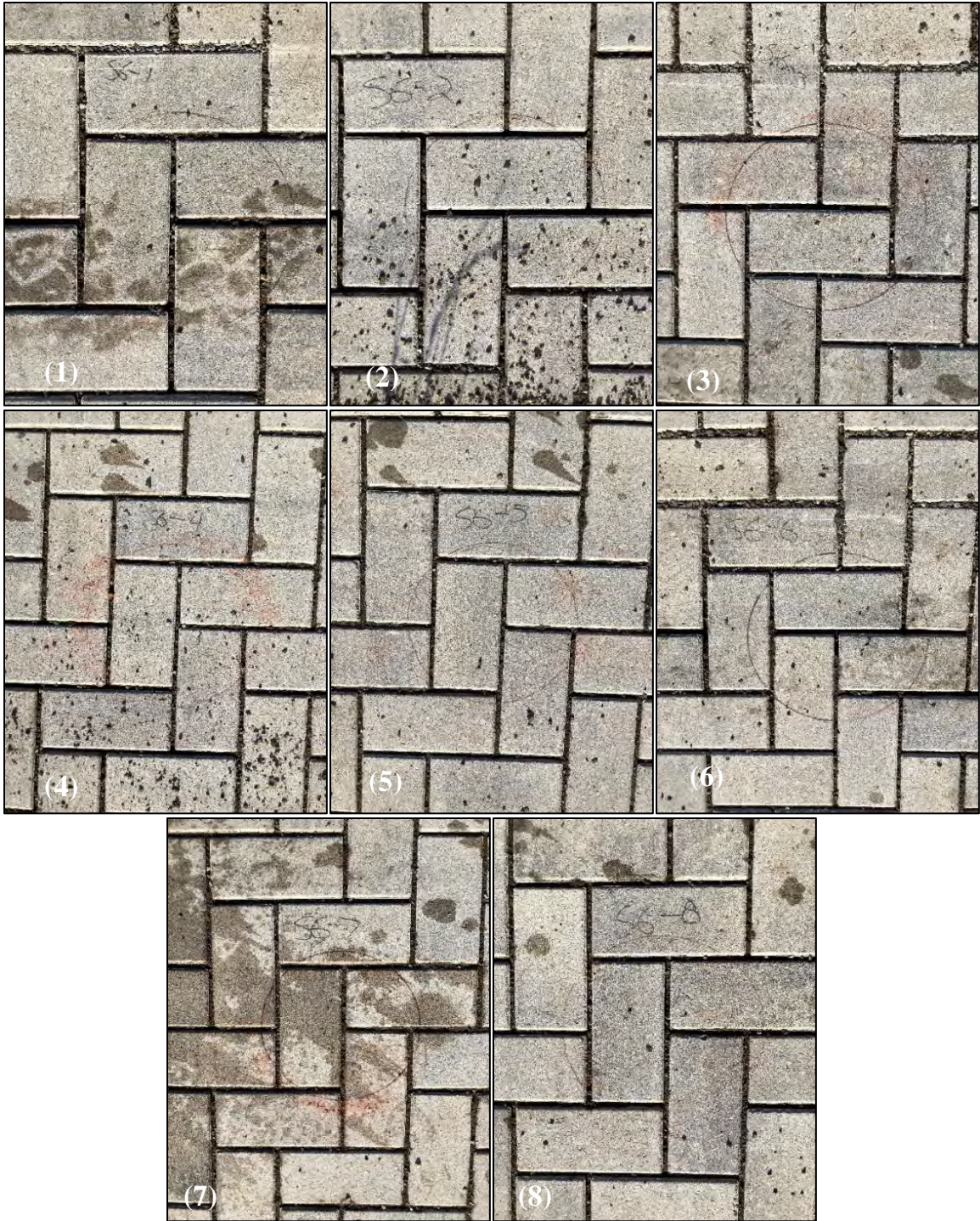
Figure J6. Post-maintenance photos of infiltration measurement locations (1-8) following a regenerative air street sweeper on Cell 6 for third early and repeated maintenance (TYMCO DST-6®).
