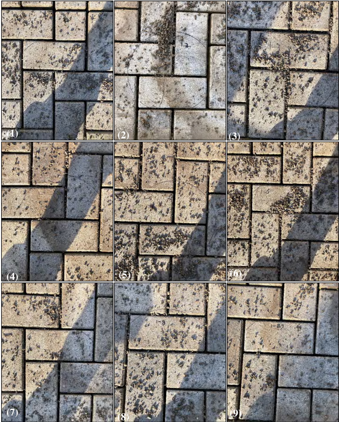
Figure I2: Post-maintenance photos of infiltration measurement locations (1-9) following high pressurized-air system on Cell 1 (Pave-Tech Typhoon®).
