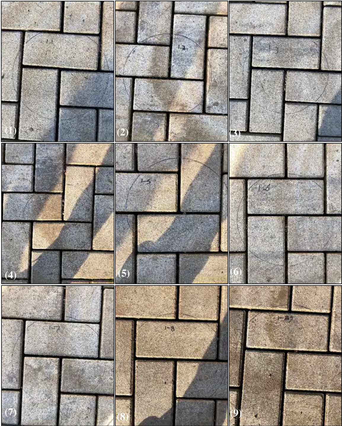
Figure I3. Post-maintenance photos of infiltration measurement locations (1-9) following a vacuum system on Cell 1 (Pavevac®).
