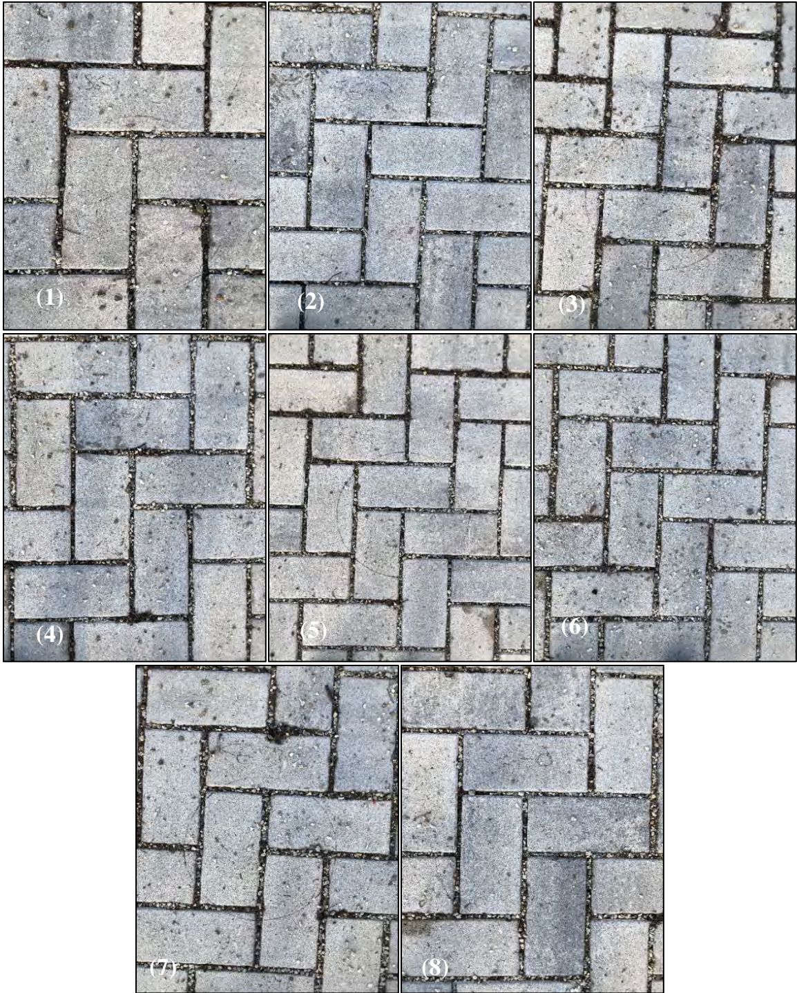
Figure J7. Pre-maintenance photos of infiltration measurement locations (1-8) on Cell 6 after third early and repeated maintenance (TYMCO DST-6®).
