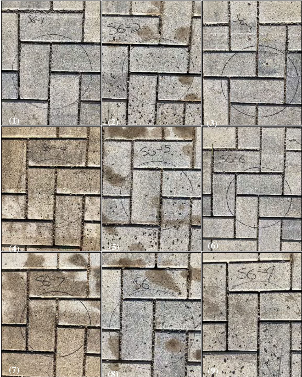
Figure J4. Post-maintenance photos of infiltration measurement locations (1-9) following a regenerative air street sweeper on Cell 6 for second early and repeated maintenance (TYMCO DST-6®).
