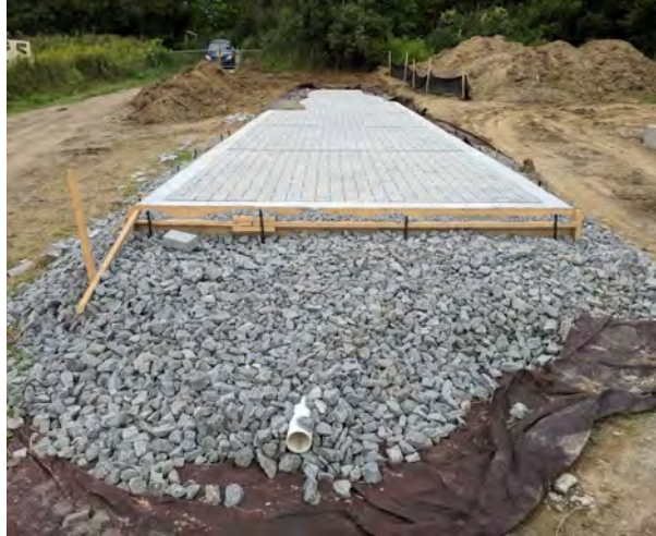
Figure 2-2: Test pad following construction (Aug 18 th , 2017).
