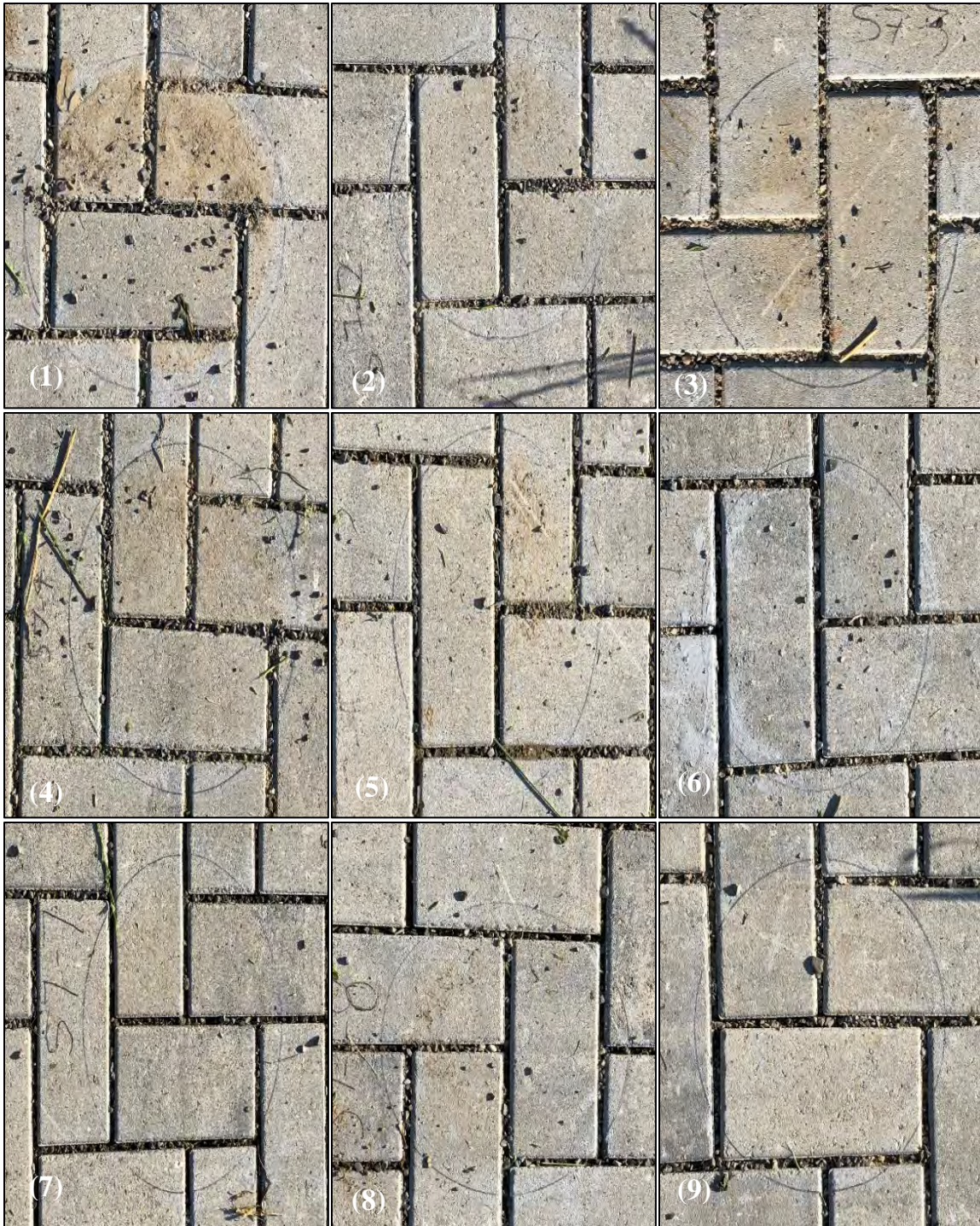
Figure K1. Pre-maintenance photos of infiltration measurement locations (1-9) on Cell 7 (Pave-Tech Typhoon® and Pavevac®).
