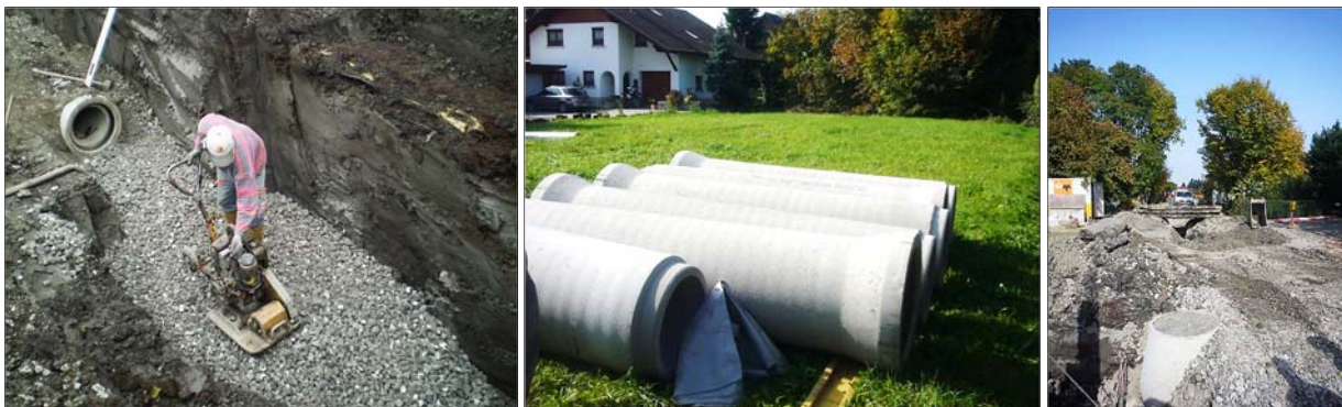
Fig. 1 Pipeline construction project, Lustenau, Austria, September 2008
