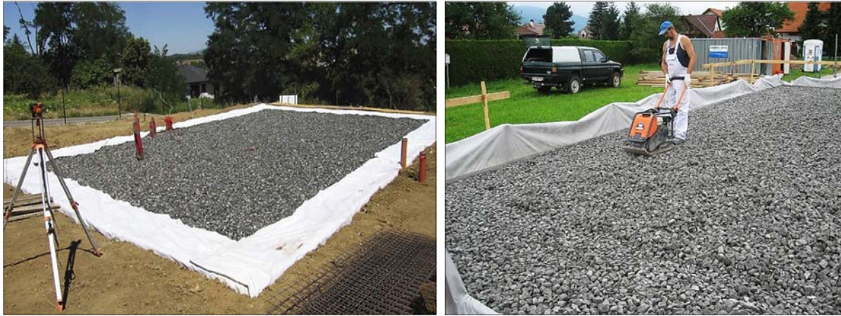
Fig. 2 Building insulation below floor slab: sub-base insulation with foam glass gravel Source: GEOCELL® foam glass gravel
