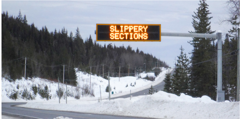
Highway 97 Variable Message Sign controlled by Highway Hush Lake Road Weather Station
