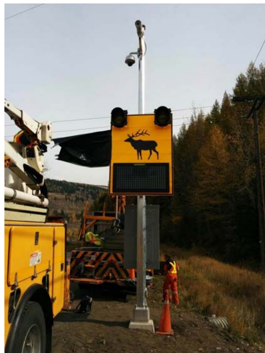
Figure 6. Installing wildlife detection system and warning signs at Michel site
