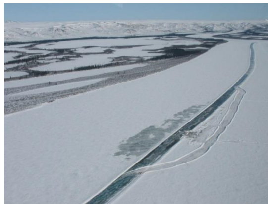
Figure 3: On-ice segment of the Inuvik-Tuktoyaktuk winter road in the NWT (Photo: A. Barker, April 18, 2012) – a by-pass was set up to go around a breakthrough.
