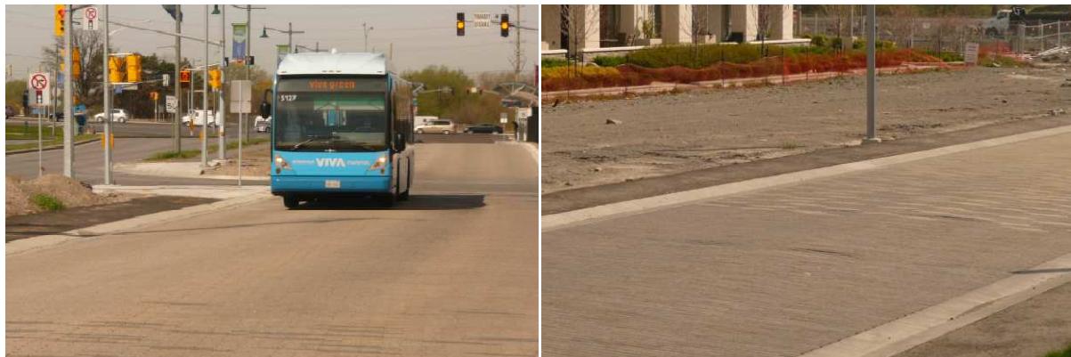
Figure 6 – Surface with Paving Bricks looking away from the Sun (left) and in the direction of the Sun (right)
