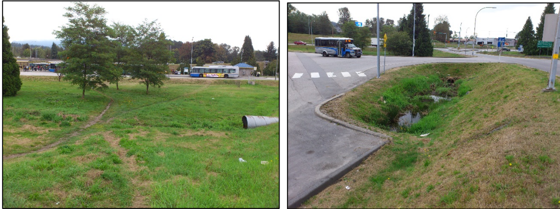
Figure 4: Existing Site Drainage and Stormwater Management
