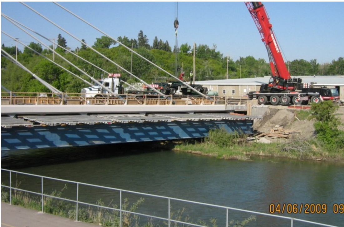
FIGURE 10 – PICTURE OF STEEL GIRDERS SUPPORTING THE FORMS.
