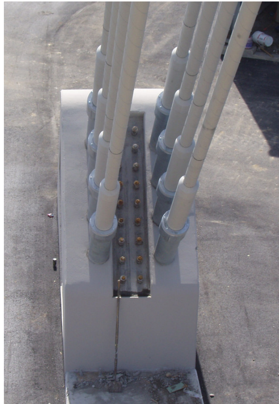
FIGURE 7 – ANCHOR BLOCK POST-TENSIONING
