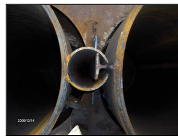
Figure 7 – Detail of Interlocking
