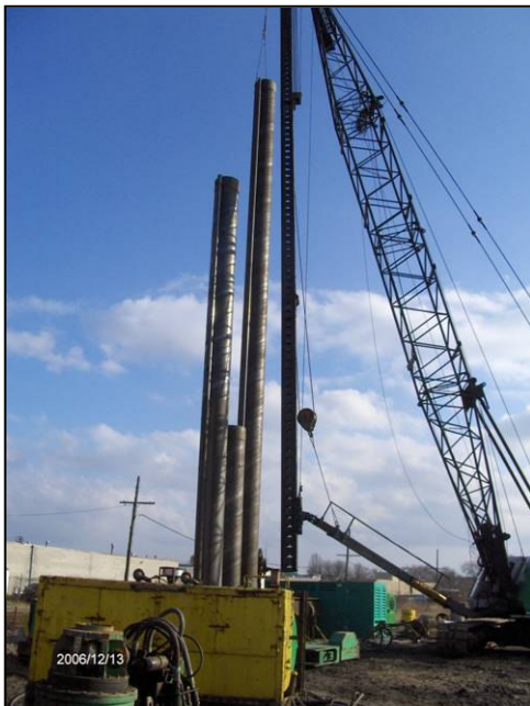
Figure 12 – Pile Demonstration at Project Site
