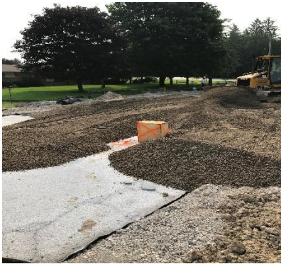
c. Placing granular A around sensors on LCC
