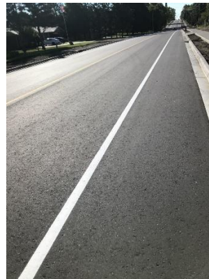
f. Completed road section
