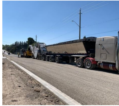
d. During asphalt paving operation
