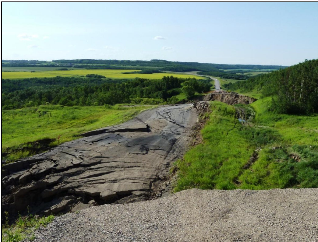
Photo 2: Damage to PTH 83 after the 2012 landslide
