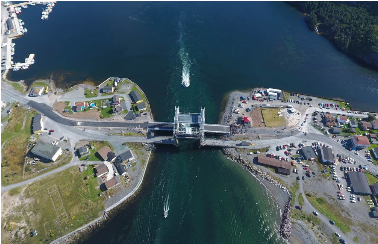
Figure 1 – Placentia Lift Bridges crossing the Placentia Gut
