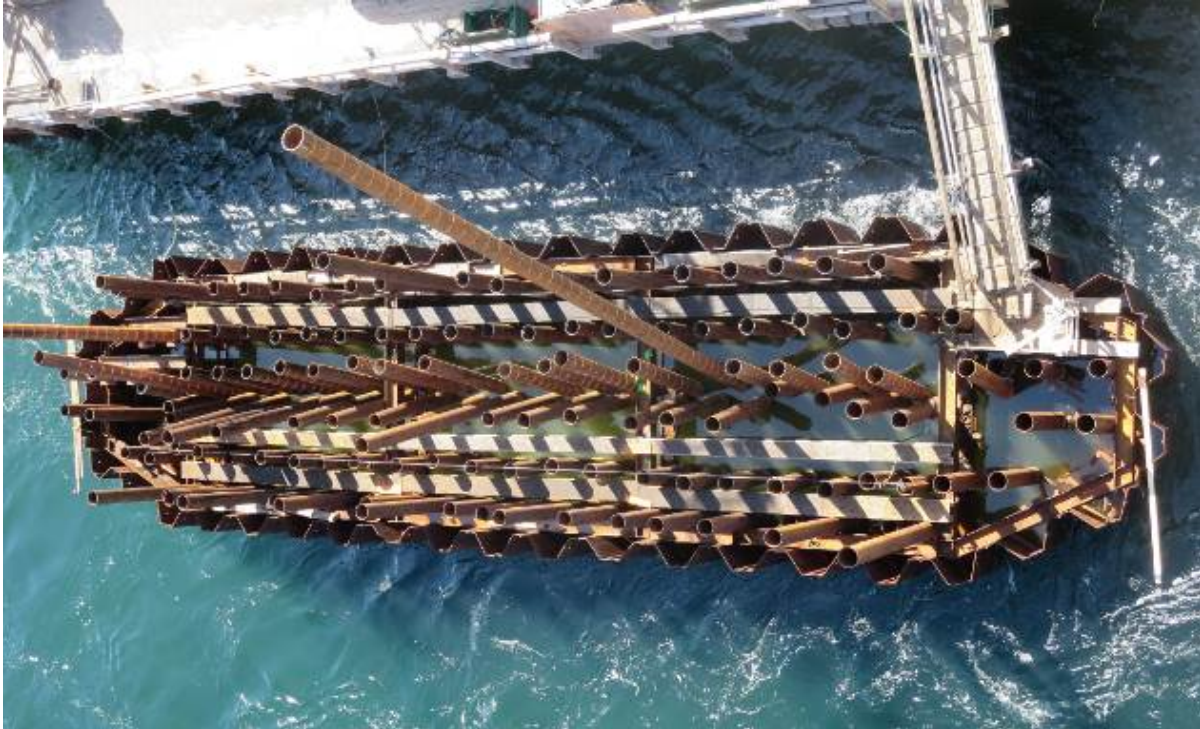
Figure 7 – Pipe piles at pier foundation
