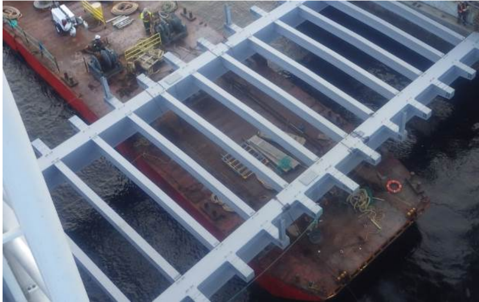
Figure 12 - Lift span framing system
