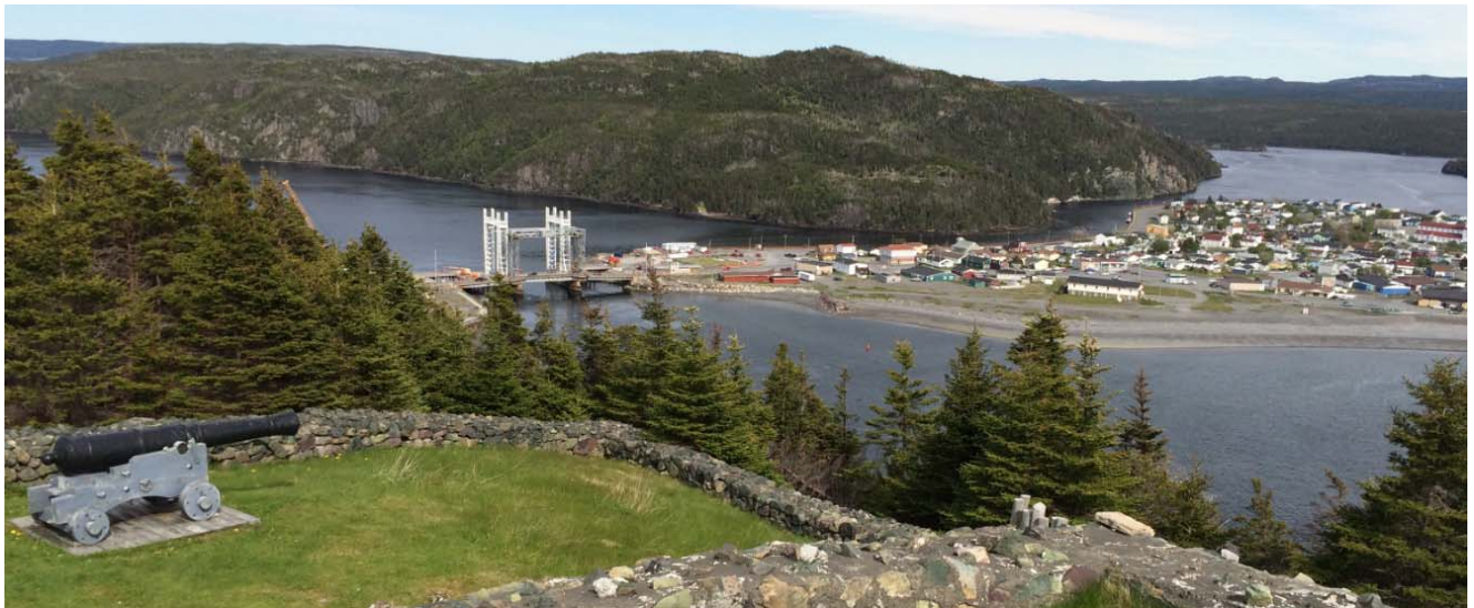
Figure 3 – View of the Bridge from Castle Hill National Historic Site
