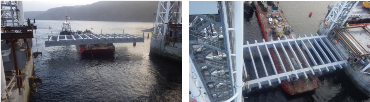
Figure 17 - Moving lift span into position
