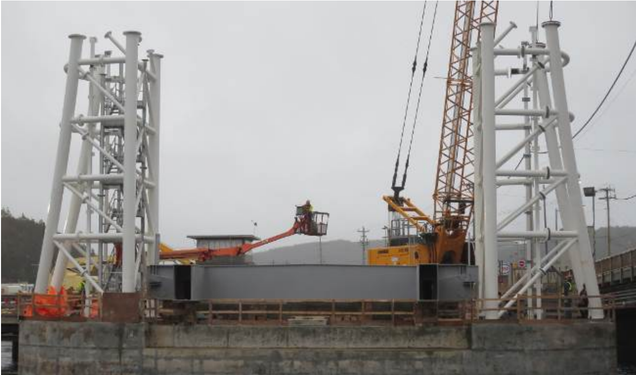
Figure 16 - Tower bolted connections
