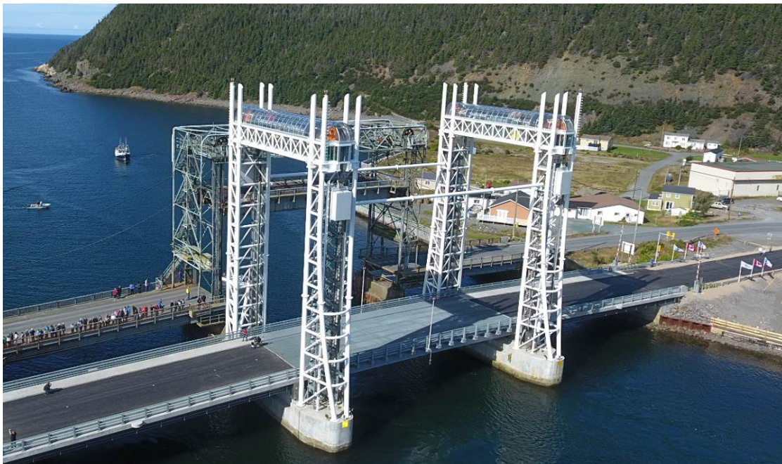
Figure 18 - Sir Ambrose Shea Vertical Bridge on opening day September 23, 2016
