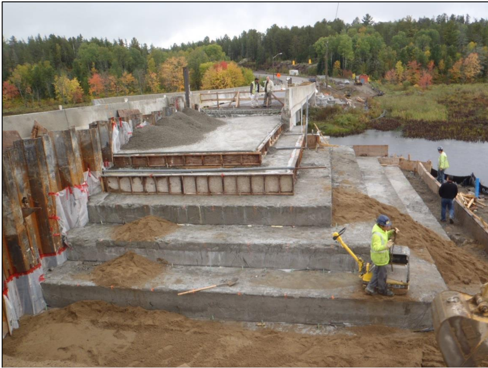
Photo 3 – Completed Northern Embankment
