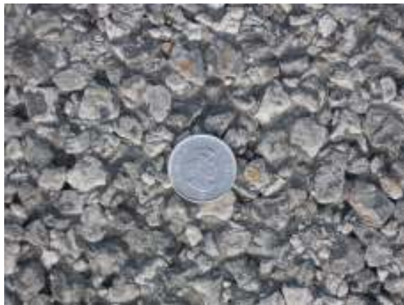
Figure 7. Stone Mastic Asphalt at CPATT-Waterloo Region Quiet Pavement Test Site
