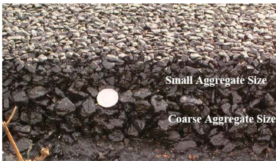
Figure 6. Double layer porous asphalt in Netherlands (21).
