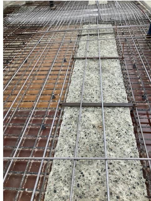
Figure 17 - Installation of new rebar
