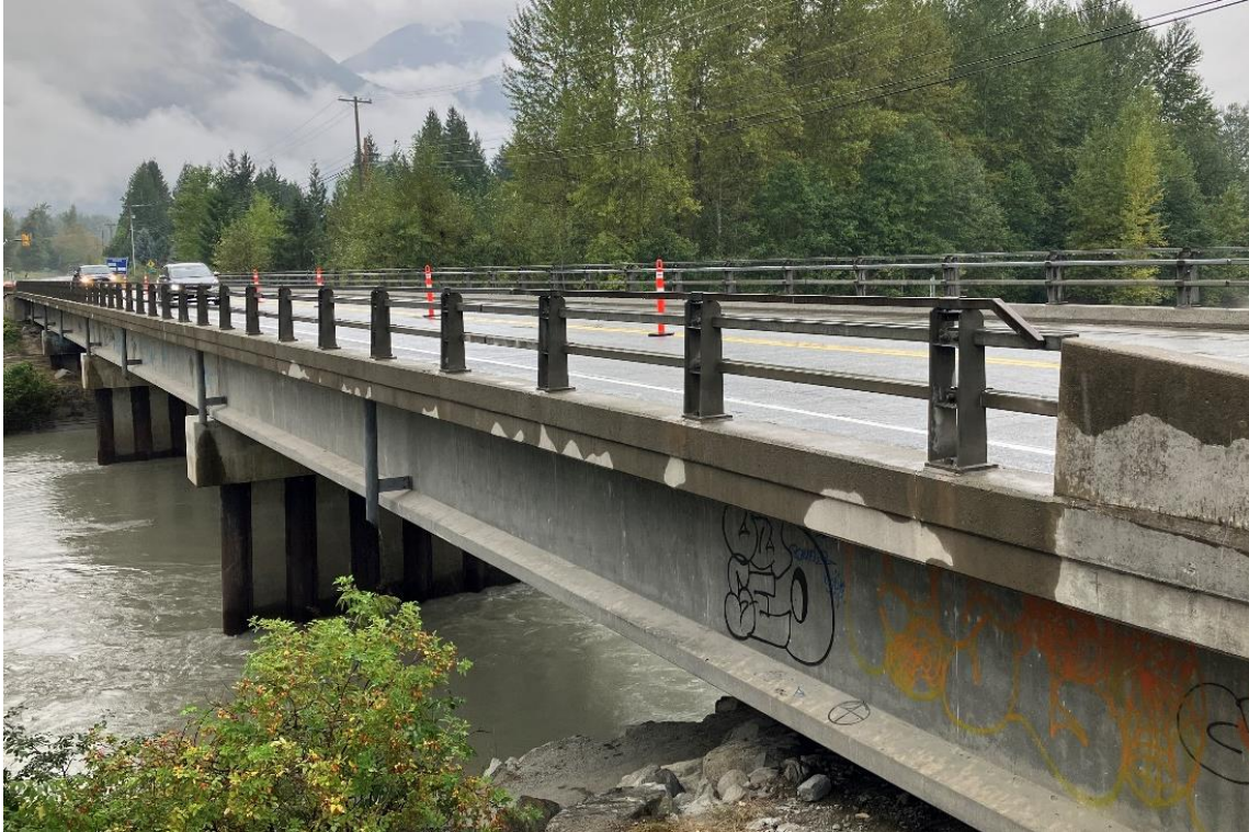
Figure 20 – Elevation view of bridge with completed new deck
