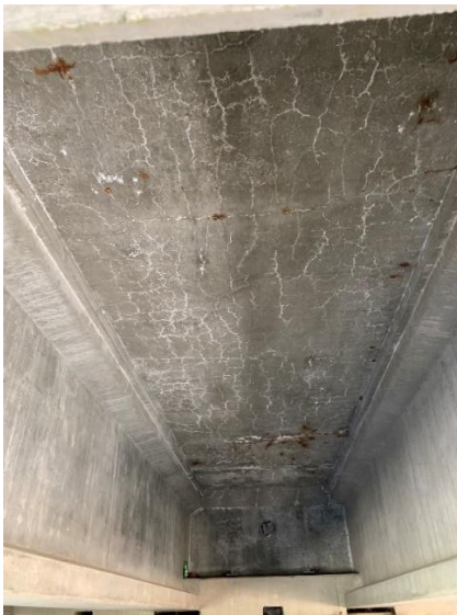
Figure 4 – (a) Area of deck soffit with deterioration (b) Crack and delaminated concrete in deck soffit
