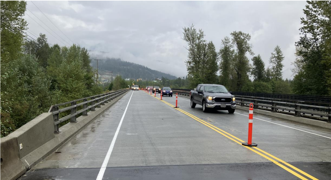
Figure 19 – Completed new deck
