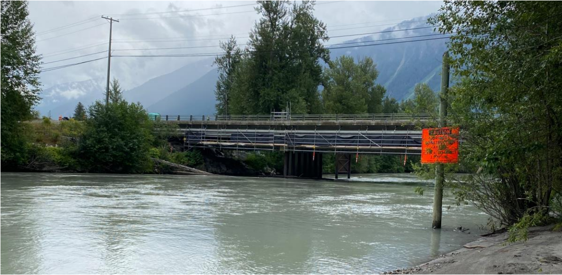
Figure 18 – Suspended scaffolding over water (orange sign showing vertical clearance)
