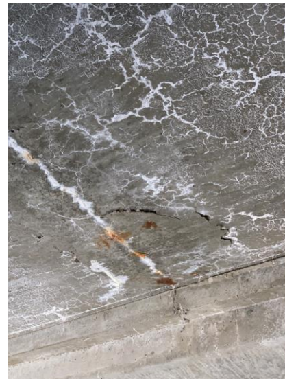
Figure 4 – (a) Area of deck soffit with deterioration (b) Crack and delaminated concrete in deck soffit
