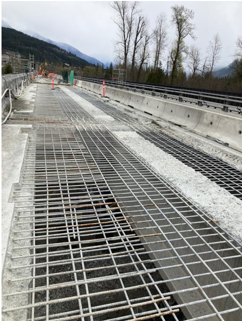
Figure 16 - Full depth concrete removed
