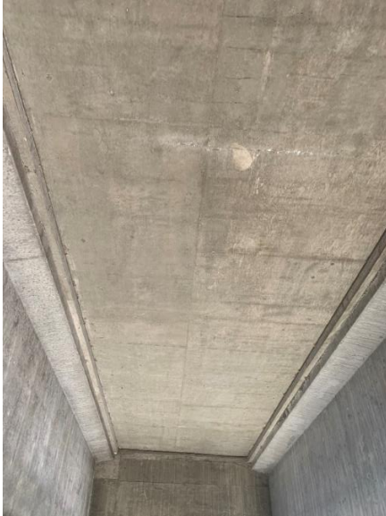
Figure 5 – Area of deck soffit with good condition
