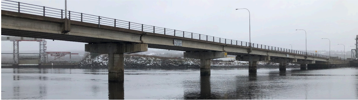
Figure 2. Existing Approach Channel Bridge
