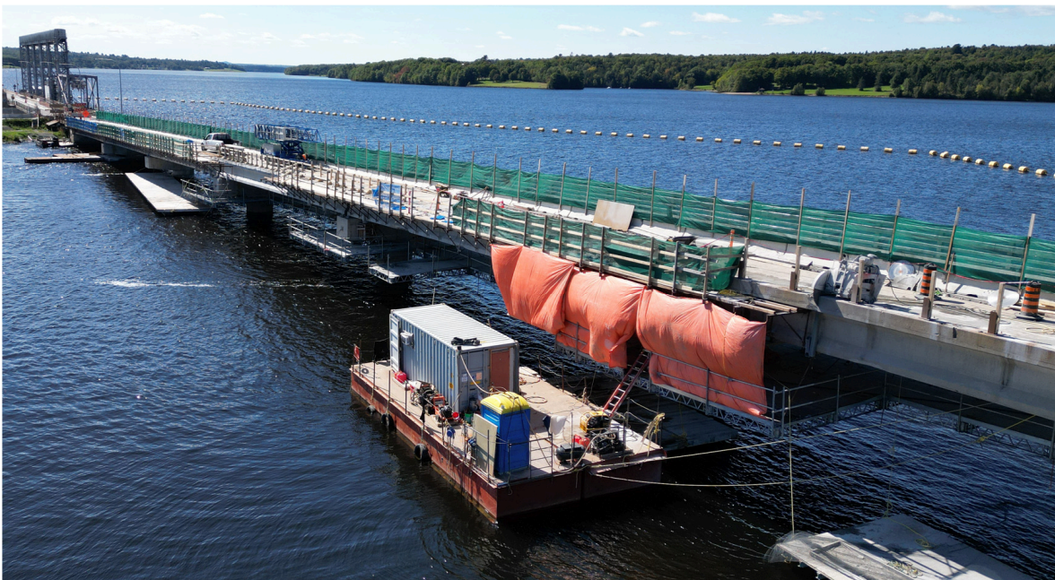
Figure 22. East half of deck asphalt and barrier partially removed.
