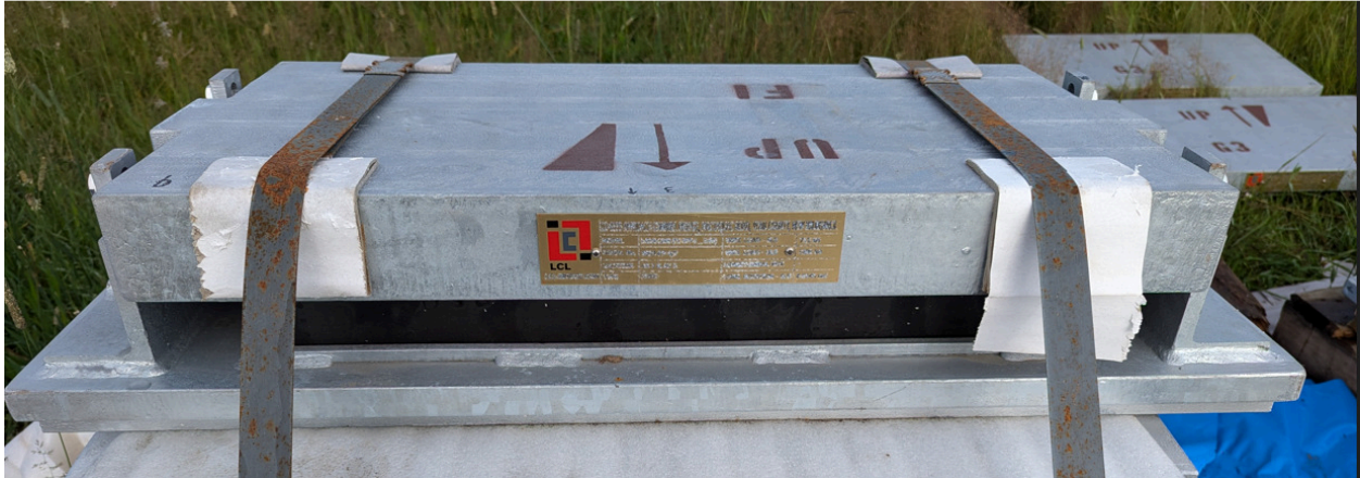
Figure 19. New bearing assemblies have been fabricated and delivered to site.
