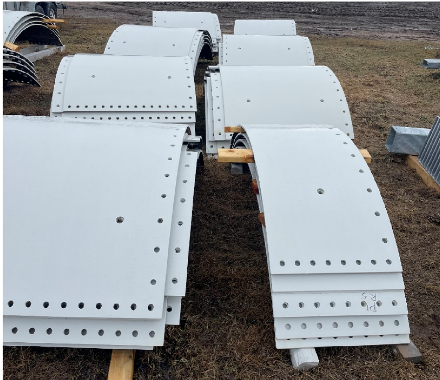
Figure 20. Coated upper pier shaft casing plates have been delivered to site and await installation.
