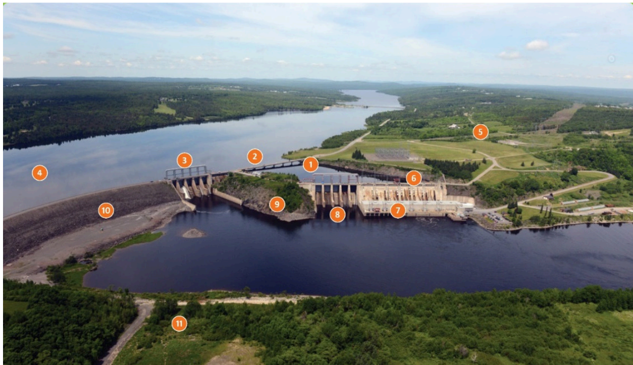
Figure 1. Mactaquac Hydroelectric Generating Station (1) Approach Channel, (2) Approach Channel Bridge, (3) Diversion Sluiceway, (4) Head Pond, (5) Keswick Ridge, (6) Intake Structure, (7) Powerhouse, (8) Main Spillway, (9) Rock Island, (10) Embankment Dam, (11) Kingsclear
