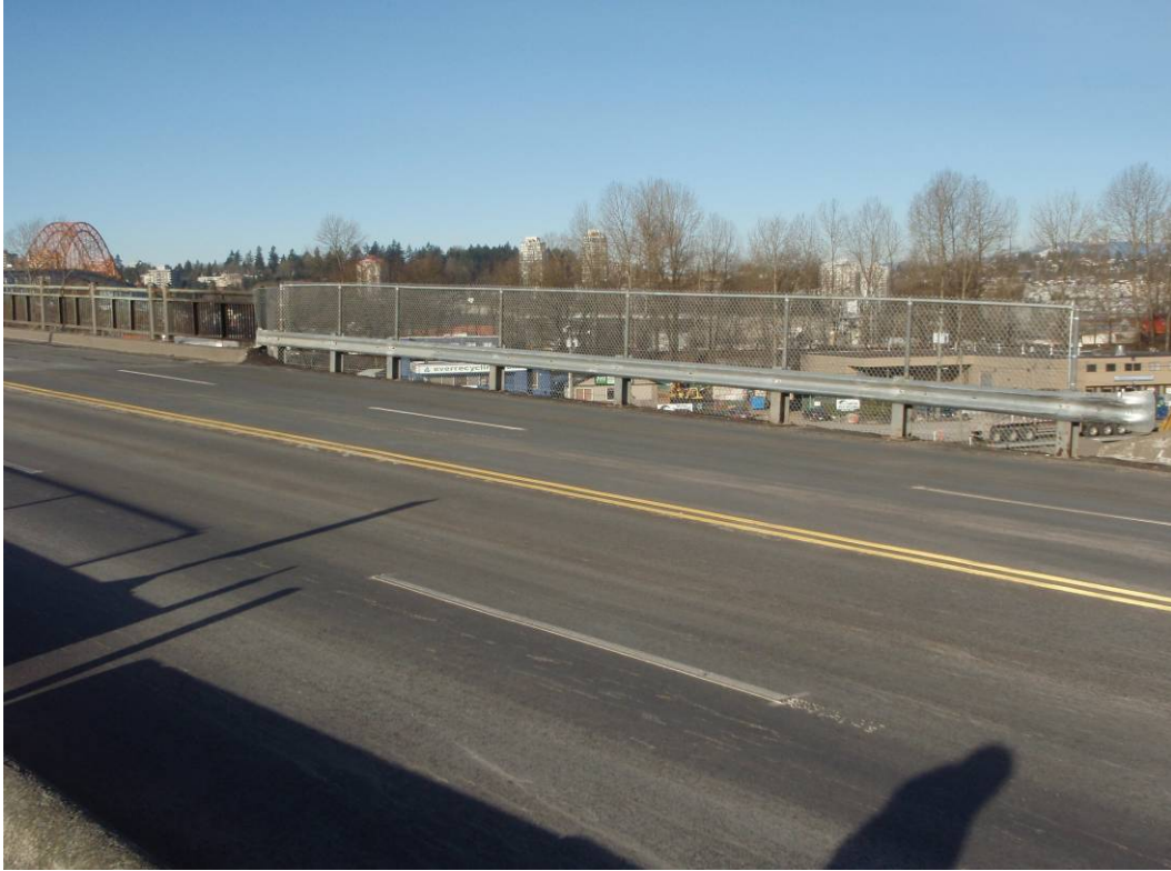
Figure 15. Completed Bridge Surface
