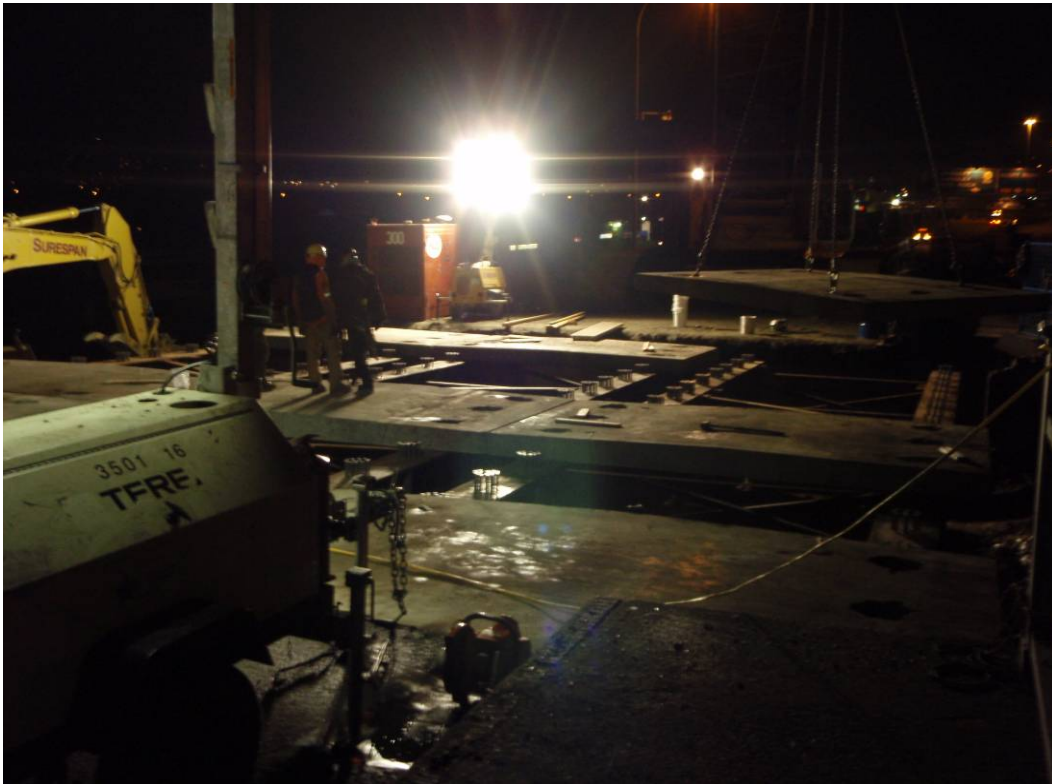
Figure 11. Work Continues through the night
