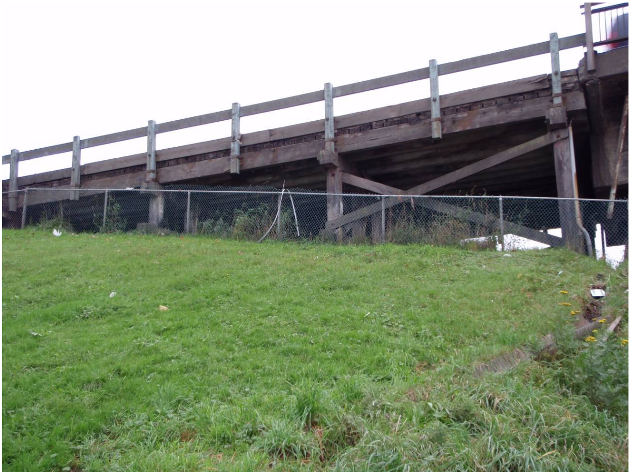
Figure 1. Undamaged Pattullo Bridge Timber Spans
