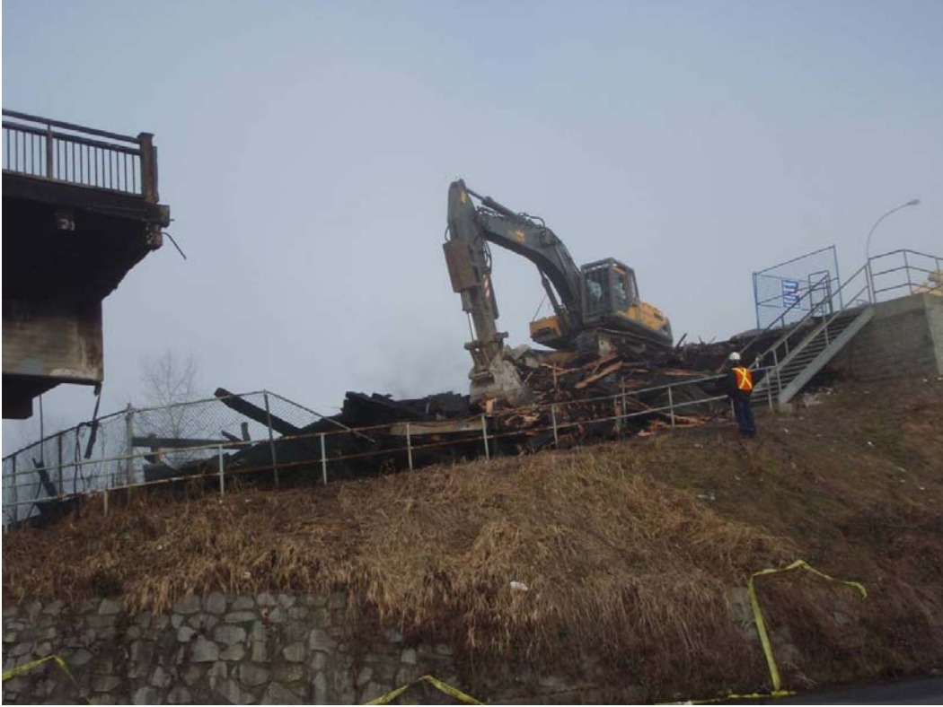
Figure 6. Demolition of Creosote Timbers
