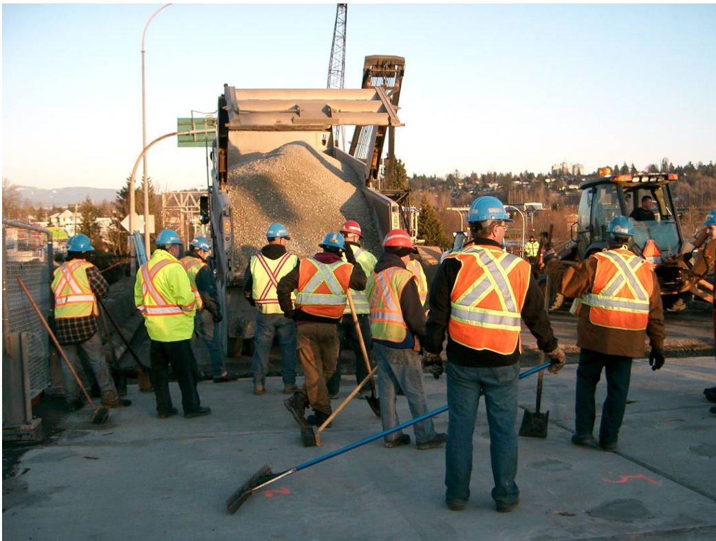
Figure 14. Backfilling and preparation for paving
