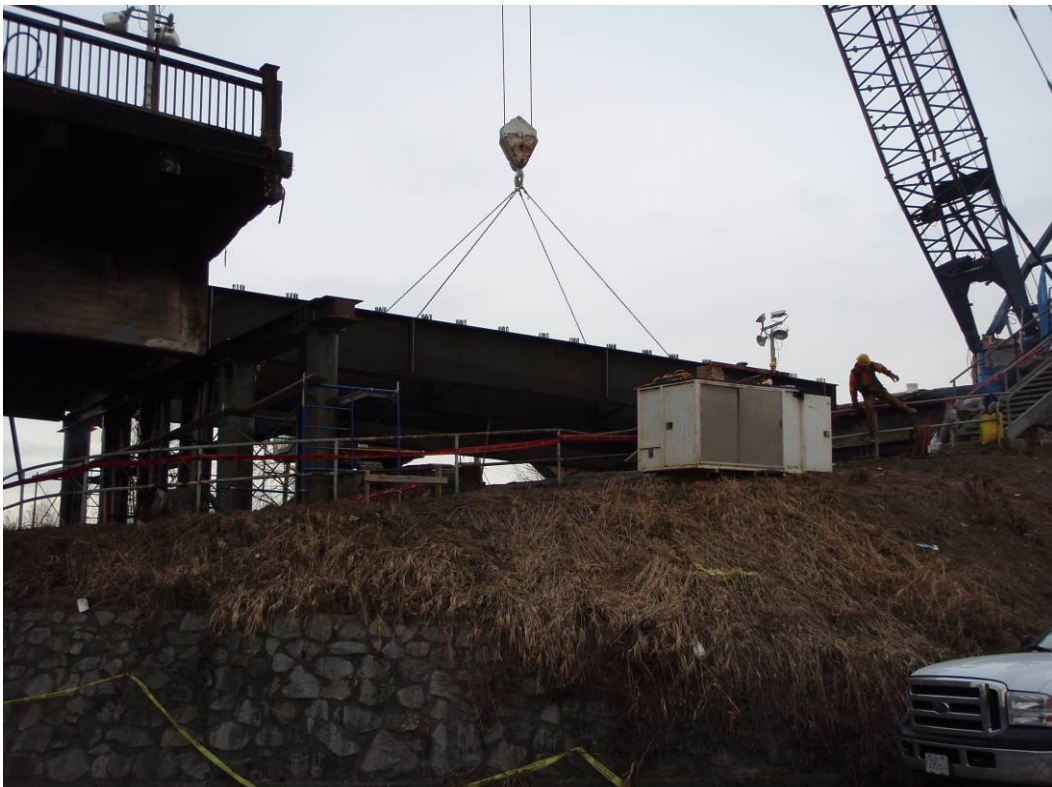
Figure 9. Erection of a Pair of Girders
