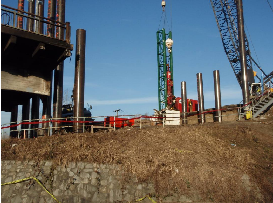
Figure 8. Pile Driving Underway
