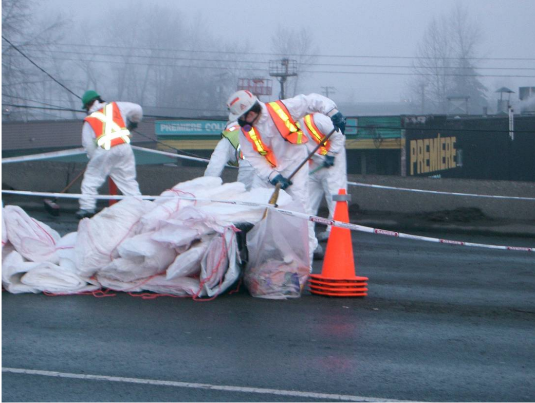
Figure 4. Specialized Person Protection for Demolition of Asphalt
