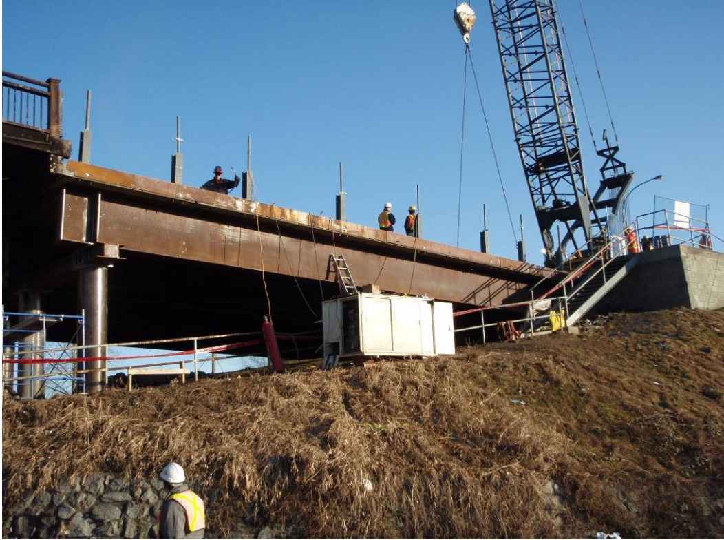
Figure 12. Installation of Railing
