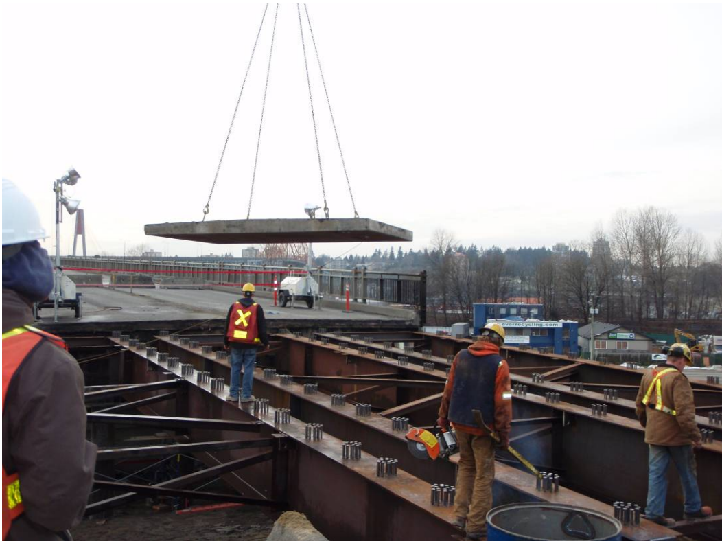
Figure 10. Erection of a deck panel
