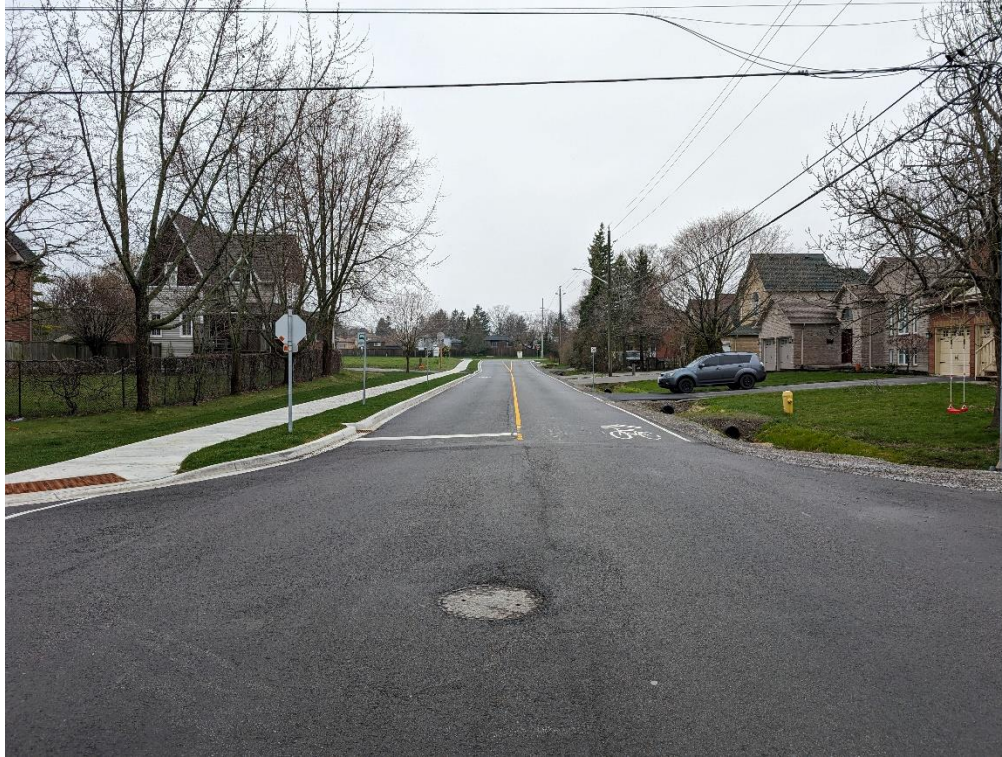
Figure 11. Range Line Road – Post Construction
