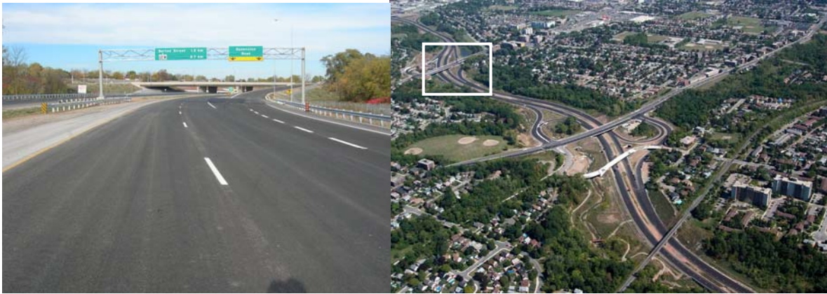
Photograph 9. Completed perpetual pavement on the Red Hill Valley Parkway.
