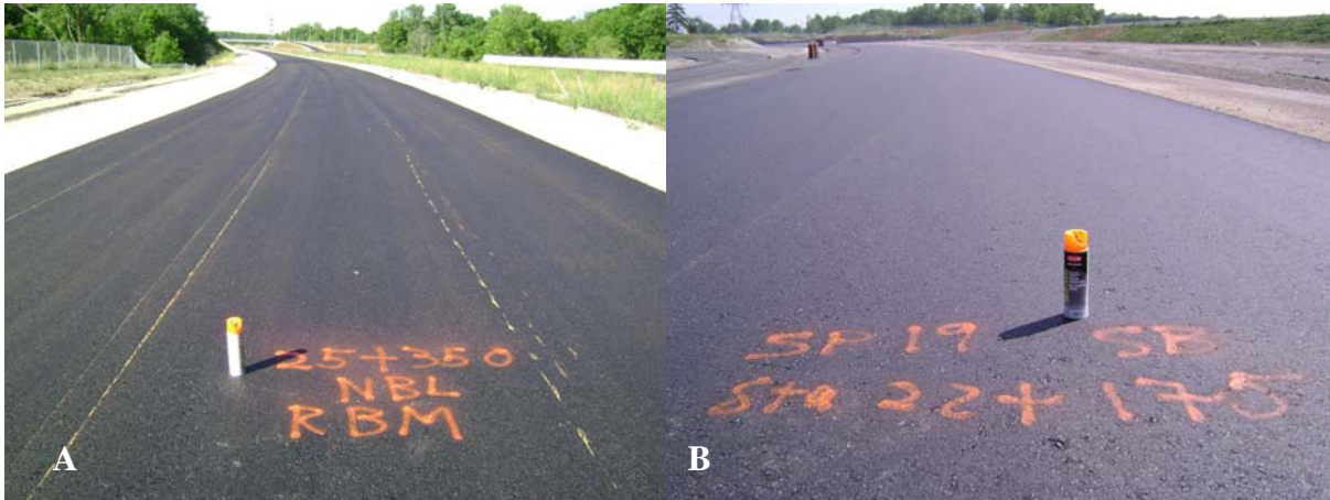
Photograph 6. Completed mats of the RBM layer (A) and Superpave 19 layer (B). No check cracking was observed after the mix adjustment.
