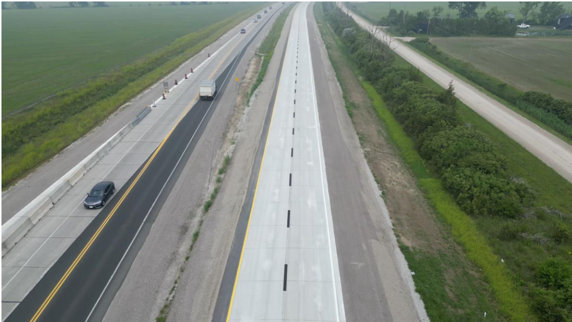
Figure 1: Aerial view of Concrete Pavement Section on Highway 3.
