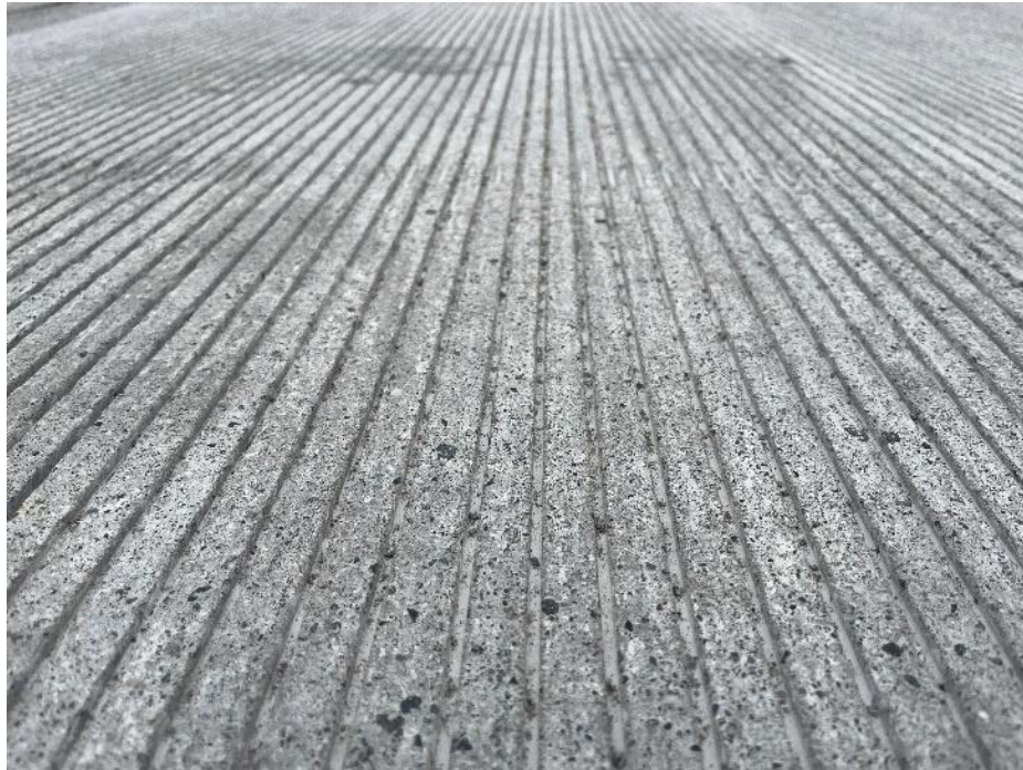
Figure 4: Close-up of longitudinally grooved concrete pavement surface on the Highway 3.
