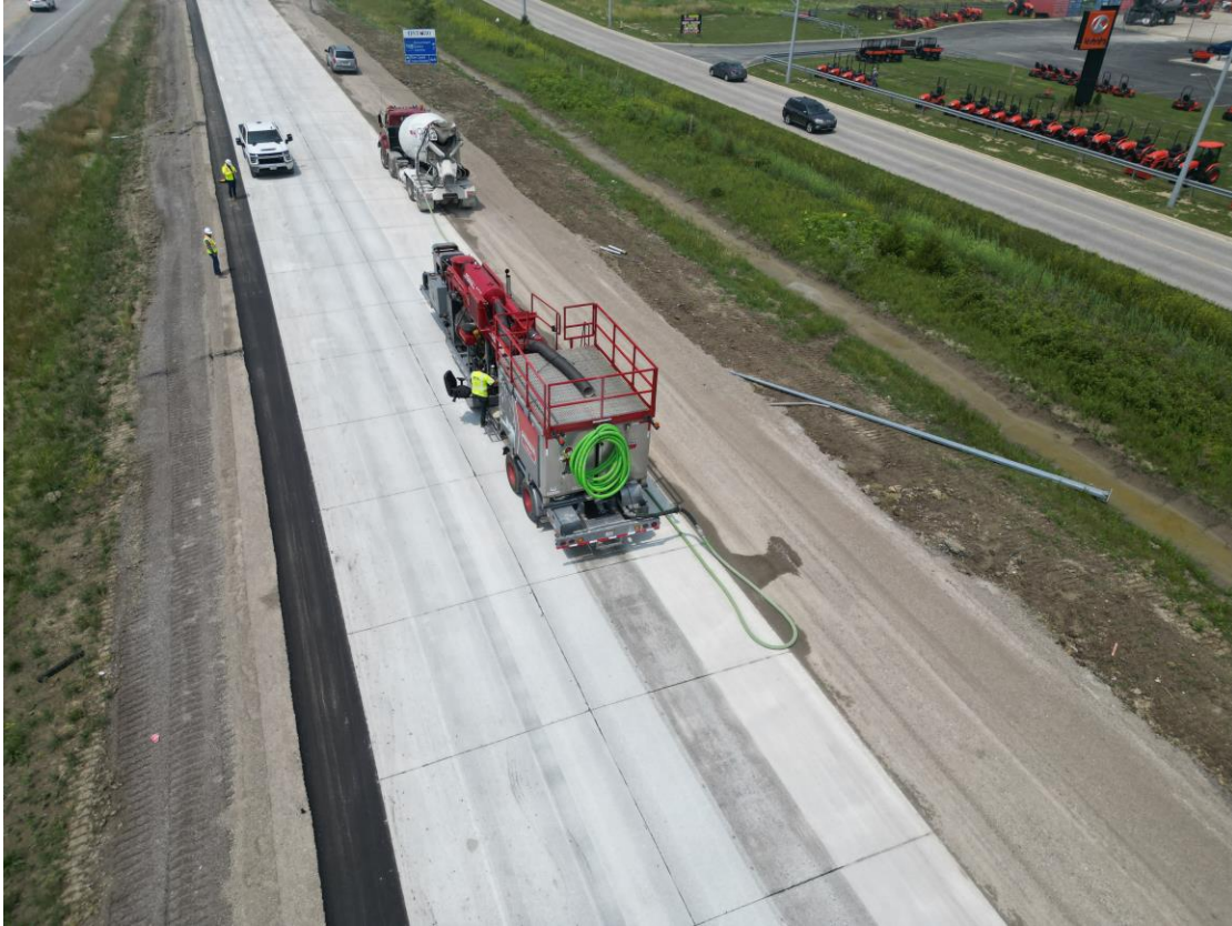
Figure 5: Diamond Grinding Operations with Ready-Mixed Concrete Truck collecting Slurry.
