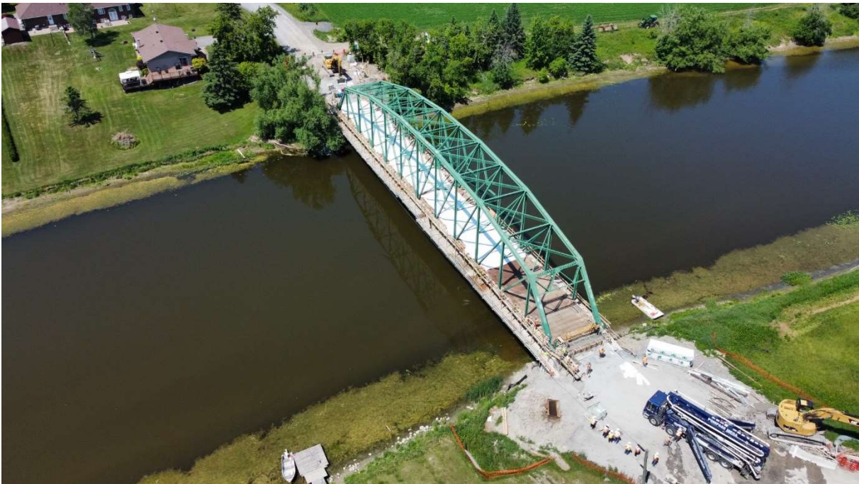
Figure 22. Aerial View of Touchette Bridge
