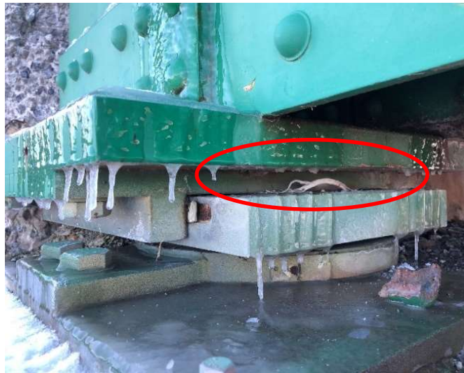
Figure 5. Dislodged PTFE at South Bearings
