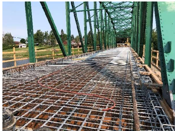
Figure 20. Stage 4 – Deck Reinforcing
