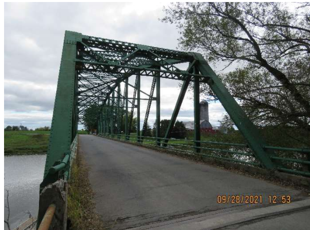
Figure 3. Bridge Deck Looking East
