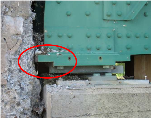
Figure 7. South Abutment Bearings in September
