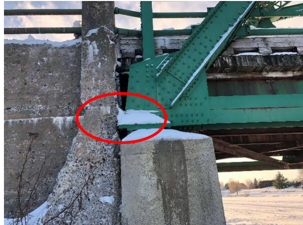
Figure 8. South Abutment Bearings in December
