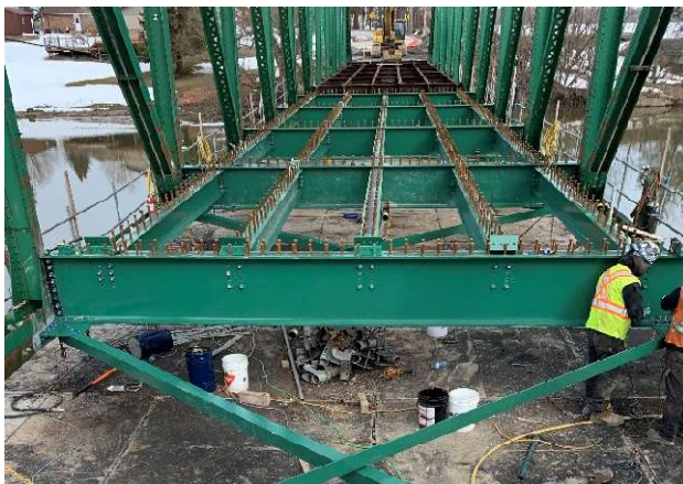
Figure 19. Stage 4 – Floor beam Replacement
