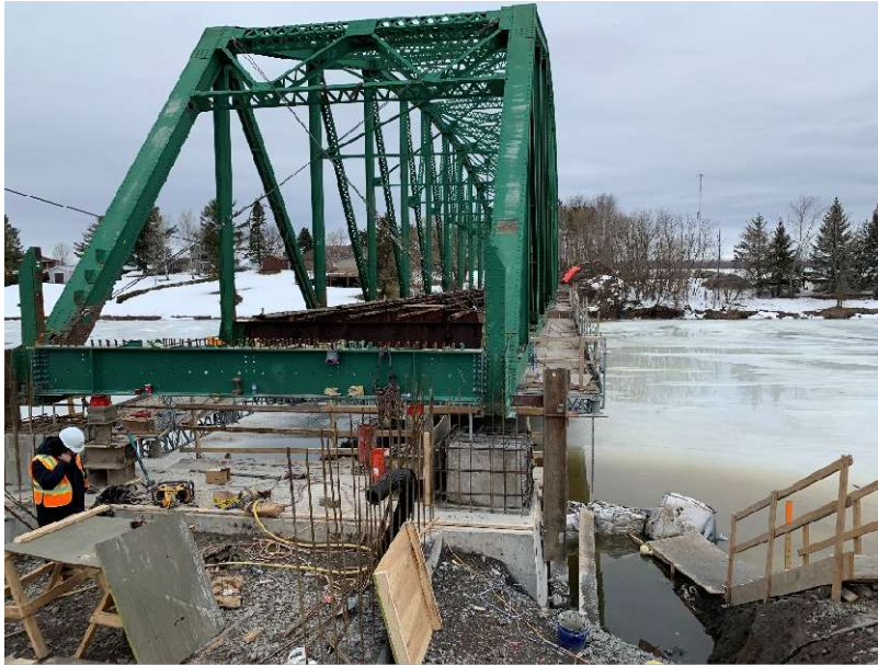
Figure 18. Stage 3 – South Abutment Bearing Replacement
