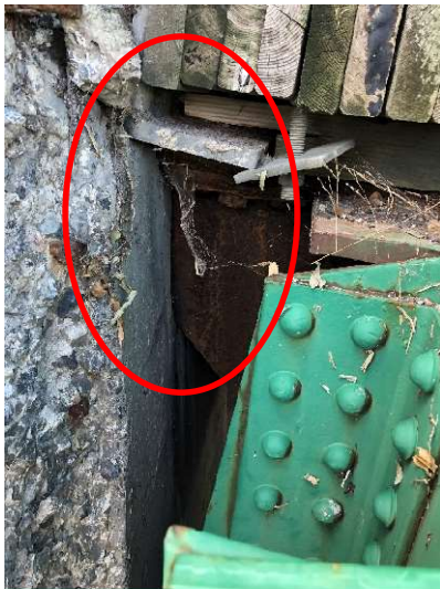
Figure 4. Truss Against South Abutment
