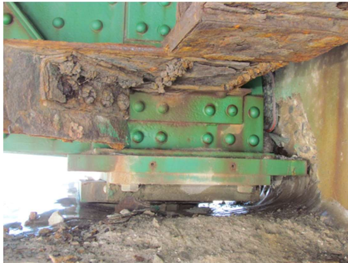
Figure 6. Superstructure Against South Abutment Ballast Wall from 2012 Winter Inspection
