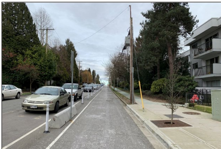
Phase 1: Quick build treatment
