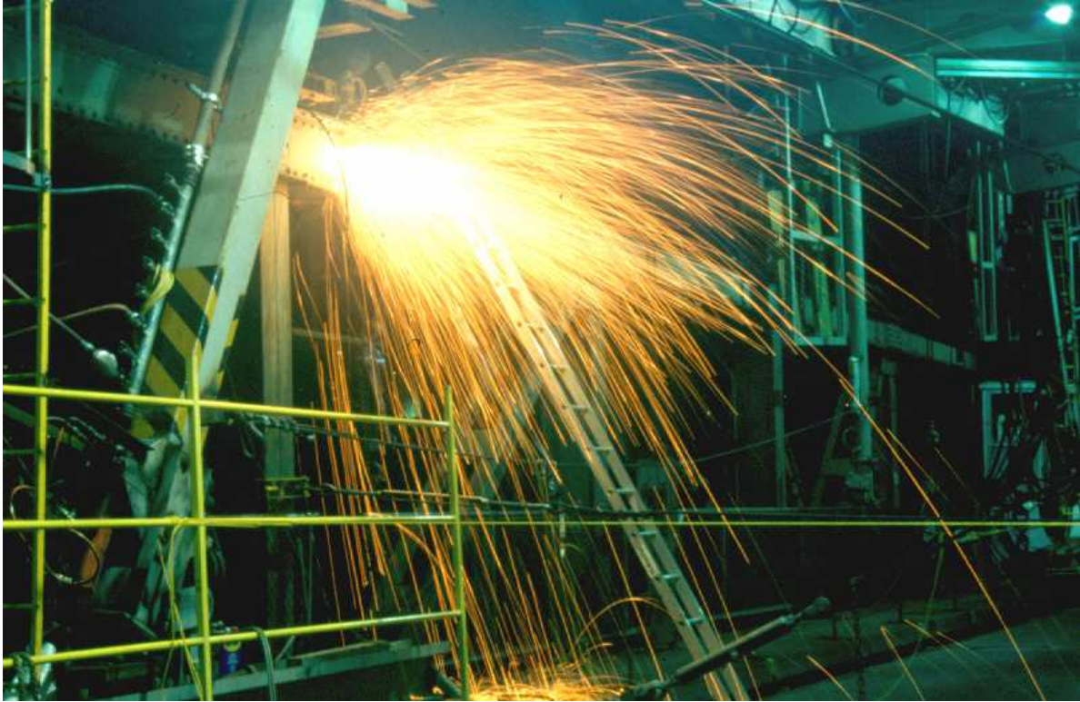
Figure 6: Cutting Old Deck Section Free
