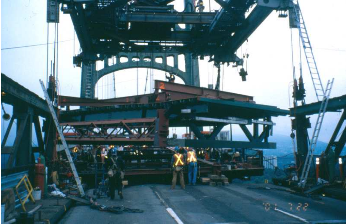
Figure 10: Modified Jacking Traveler Rotating South Side Span Section
