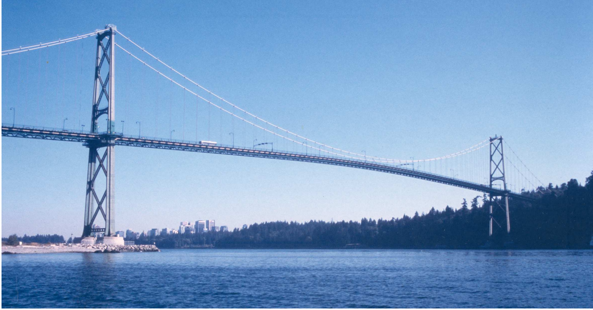
Figure 12: Overall Photo After Construction
