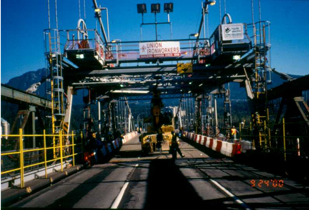
Figure 4: Contractors Jacking Traveler
