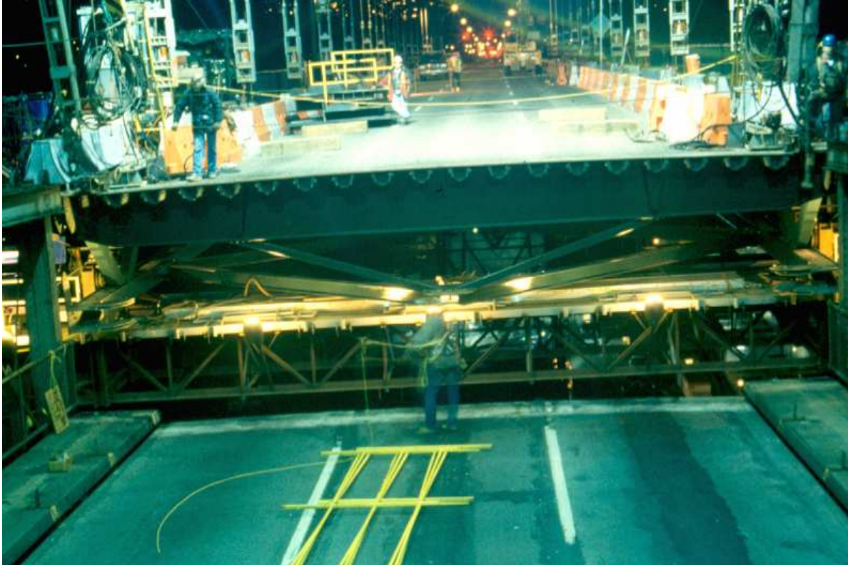
Figure 7: Lowering Old Deck Section
