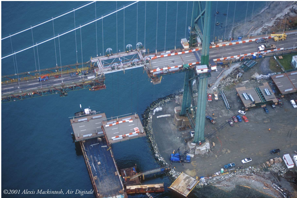
Figure 8: New Deck Section Being Raised
