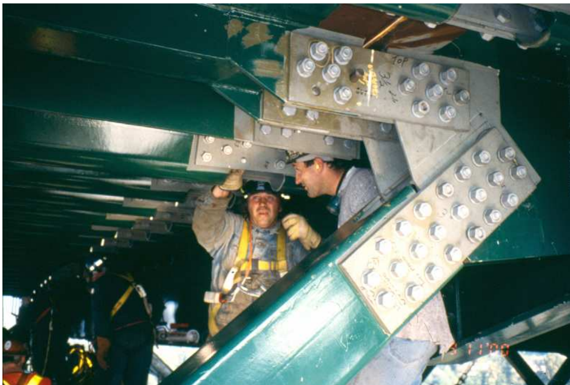
Figure 9: New Section Being Bolted to Previously Erected Section
