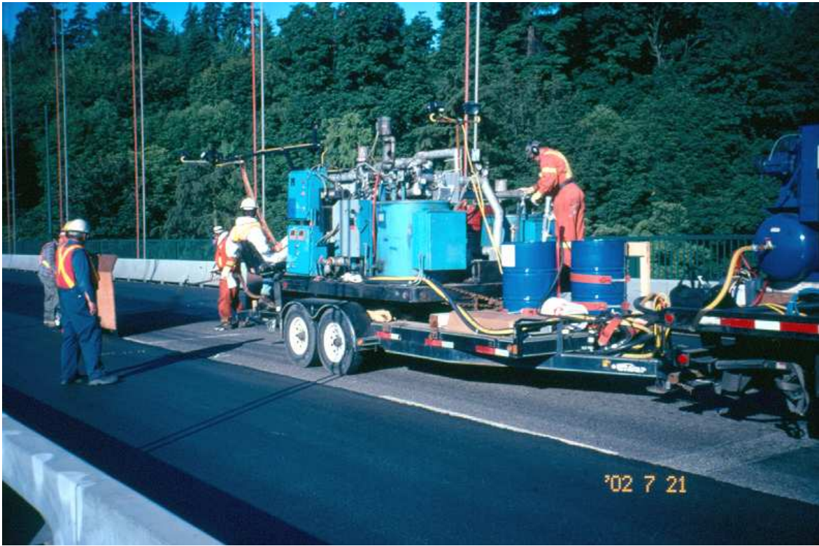
Figure 11: Final Paving Being Applied
