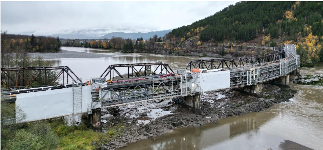
Figure 17: Coating Enclosure Work Occurring on Multiple Spans
