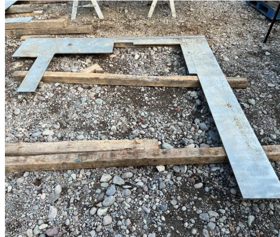
Figure 24: Steel Sheeting Cut On Site for Additional Member Repairs
