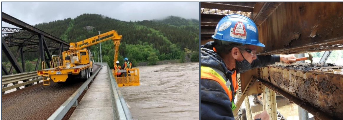
Figure 8: Snooper Truck Inspection (left) and Top Chord Inspection (right)
