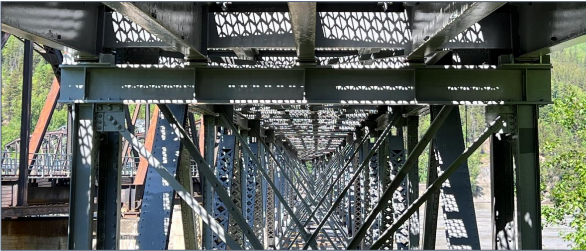
Figure 13: New South Approach Cap Beam and Elastomeric Bearings at Pier 7
