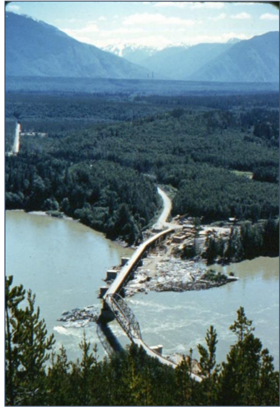
Figure 4: Widened Concrete Piers prior to Realignment to Accommodate CN Railway Bridge
