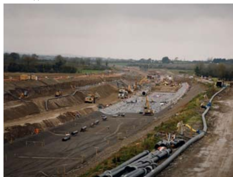
Photo 4: circulation des engins
