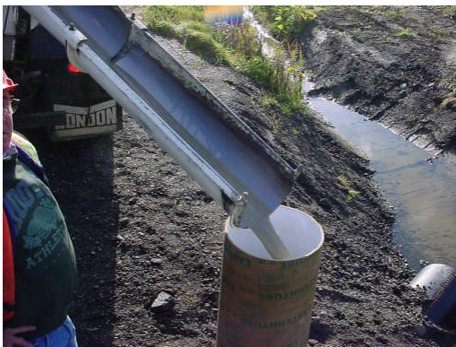
Figure 3: Grouting by gravity flow through a tube
