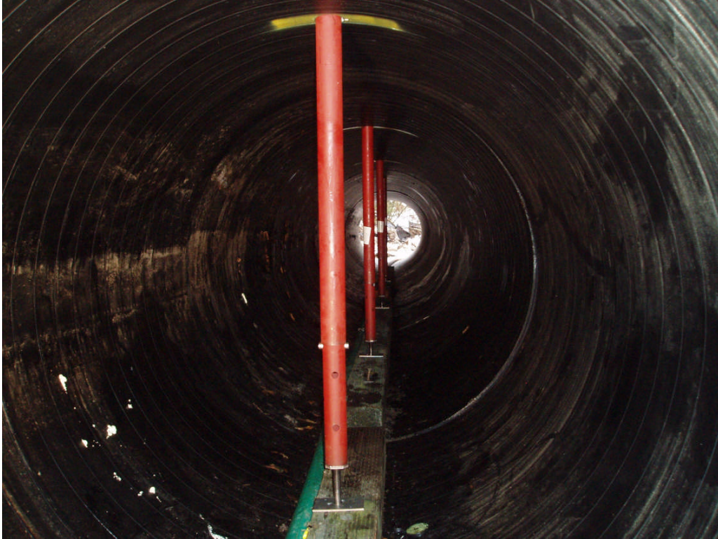
Figure 7: Temporary internal bracing during grouting operation
