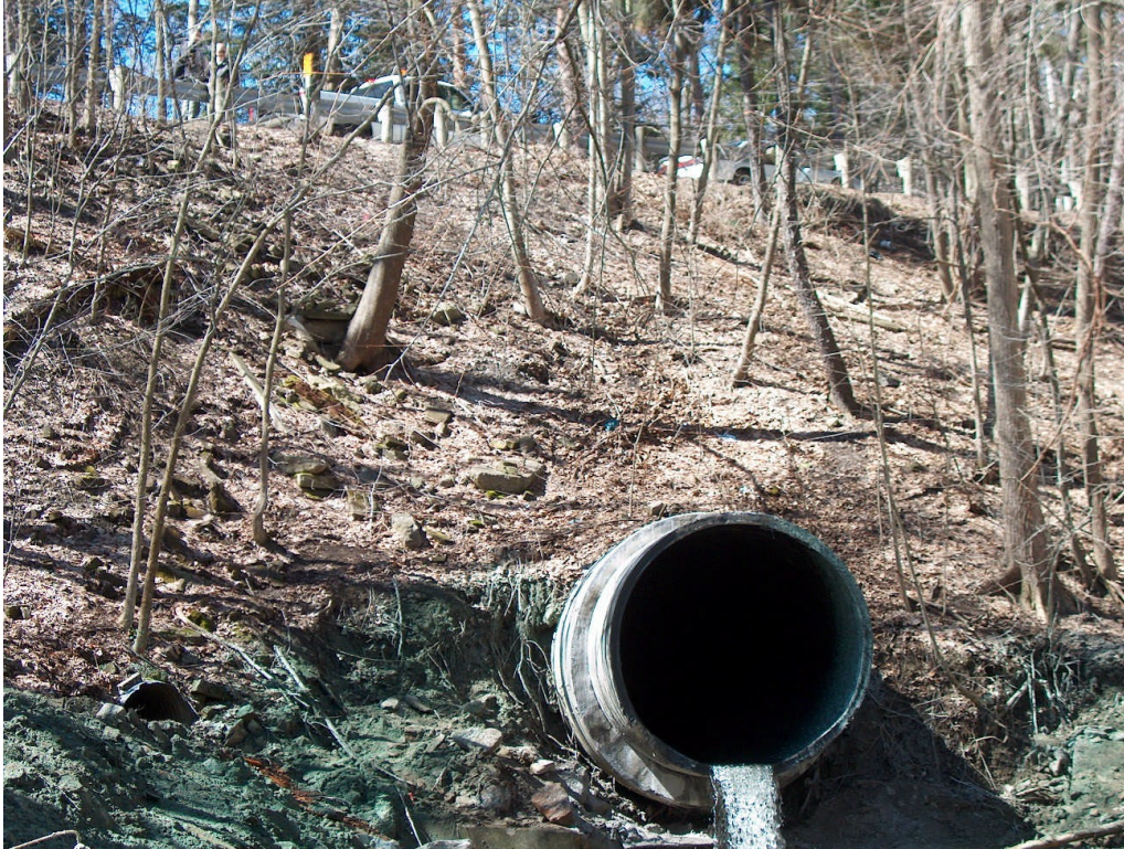
Figure 1: Culvert slipline in deep fill
