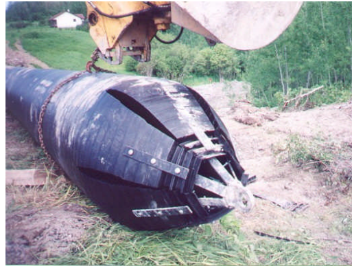
Figure 6: Field-fabricated pulling head
