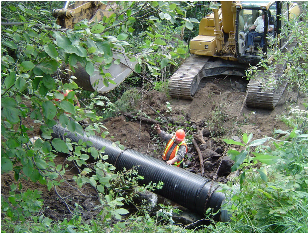
Figure 2: County of Haliburton installs Weholite® to rehabilitate an existing CMP
