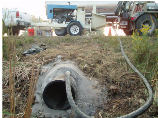
Figure 4: Pressure grouting
