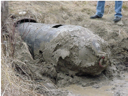
Figure 5: Fabricated mechanical pulling head
