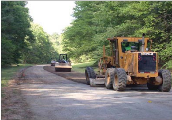
Figure 7 – Compaction and final grading.
