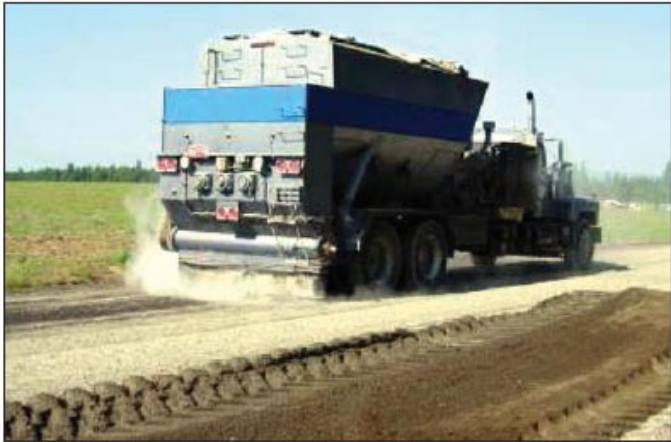
Figure 4 – Placing cement dry.
