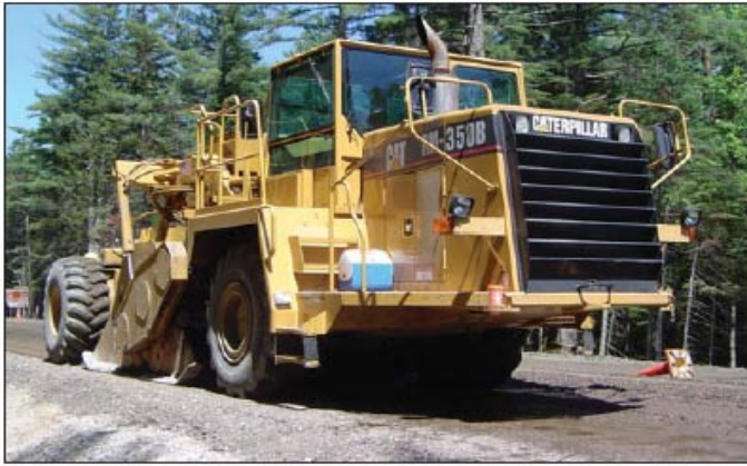
Figure 3 – Pulverizing a failed asphalt pavement.
