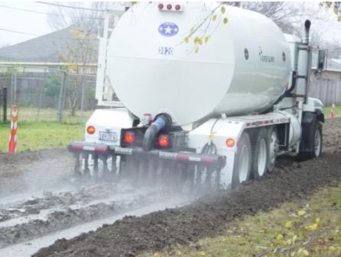
Figure 5 – Placing cement in slurry form.
