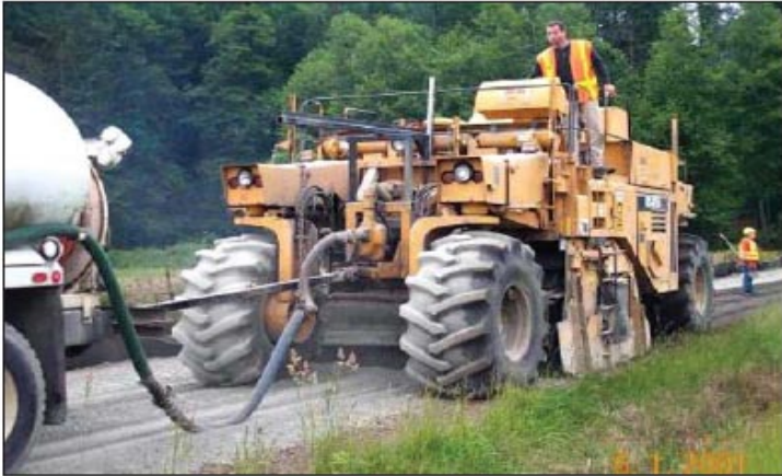
Figure 6 – Water being injected during mixing operation.
