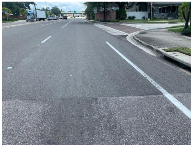
HFST on Hillsborough Ave. at Central Ave. Source: FDOT
