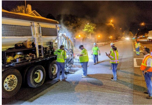
Application of HFST to Hillsborough Ave. using fully-automated installation. Source: FDOT
