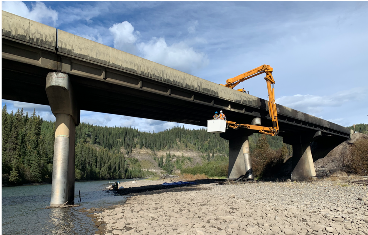
Figure 2. Spans 1, 2, and 3 of the Sikanni Chief River Bridge
