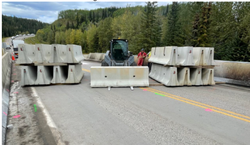
Figure 10. Static load test
