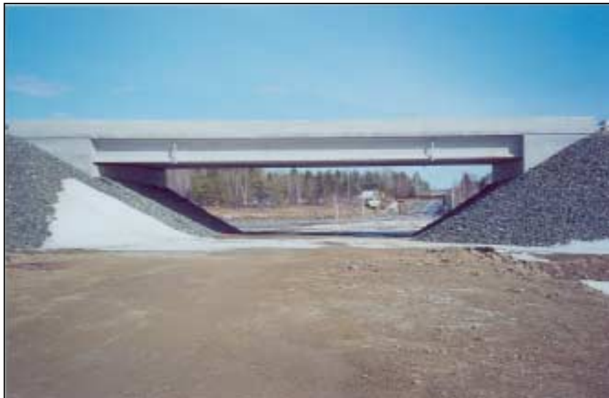
Figure 8.1: Completed overpass structure looking east
