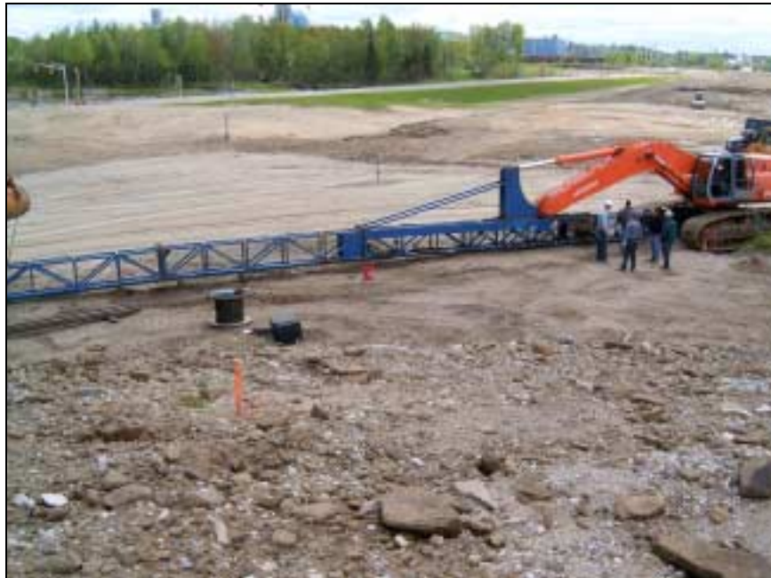
Figure 4.3: Excavator attached to mast
