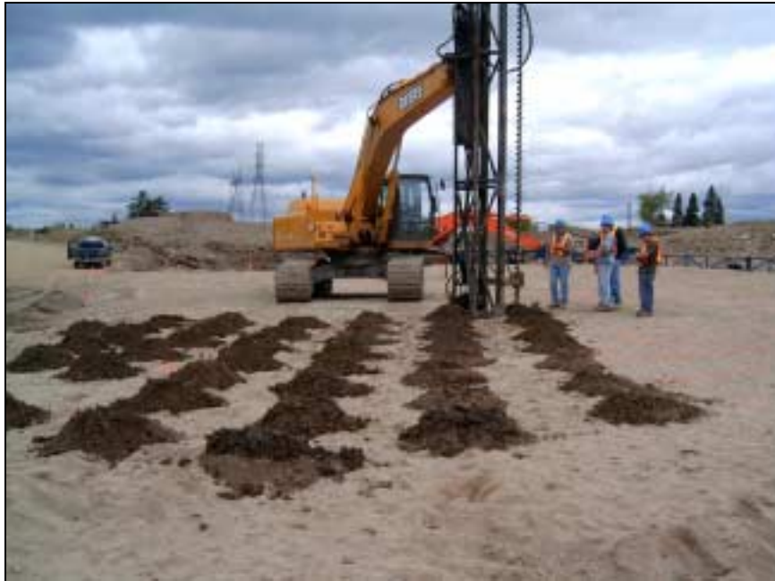
Figure 4.4: Pre-augering drain locations
