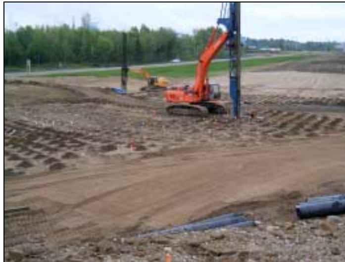
Figure 4.6: Vertical drain installation
