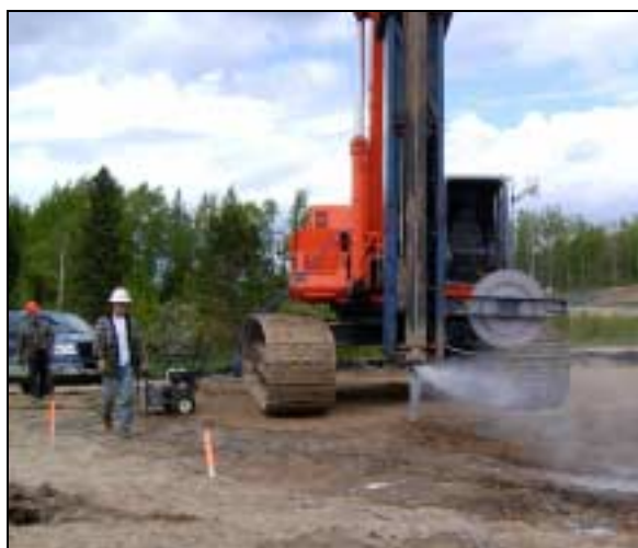
Figure 4.5: Mandrel lubrication
