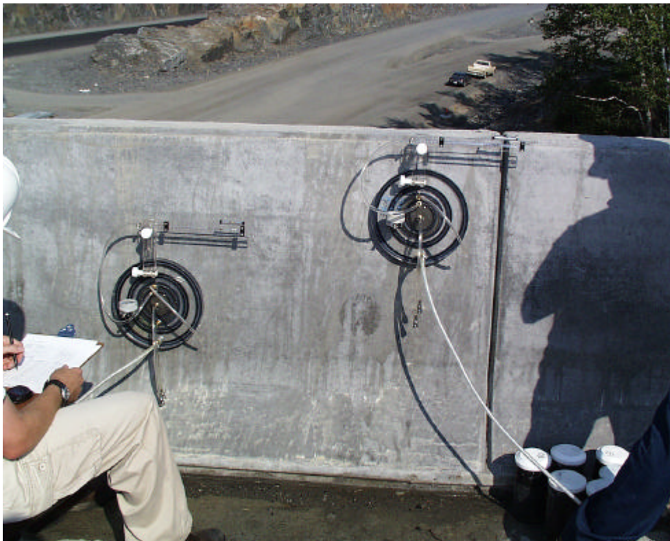
Fig.1 In-situ testing of water sorptivity, high-performance concrete barrier wall
