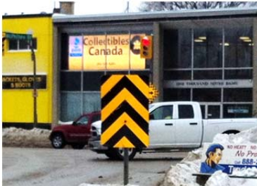
Example of a DPAD behind a traffic signal.
