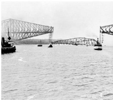
Figure 3. Collapse of the Quebec Bridge, QC, 1916 4 Library and Archives Canada
