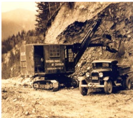
Building the Trans-Canada Highway through Glacier Park British Columbia Transportation and Infrastructure
