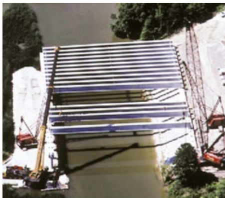
Figure 5. Highway 407 bridge over the Humber River, Toronto. After being erected the precast concrete girders, pretensioned for handling, were continuously post-tensioned from abutment to abutment for structural efficiency Canadian Precast Concrete Institute
