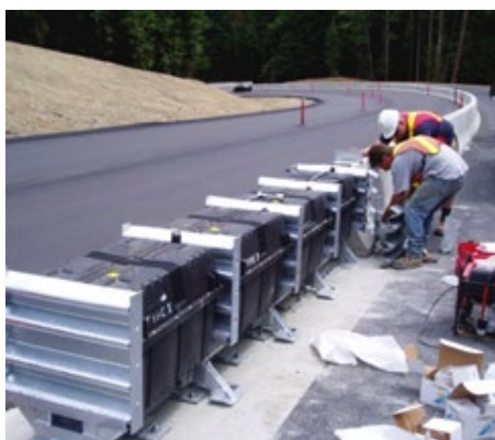
Metal Crash Barrier Installation British Columbia Transportation and Infrastructure
